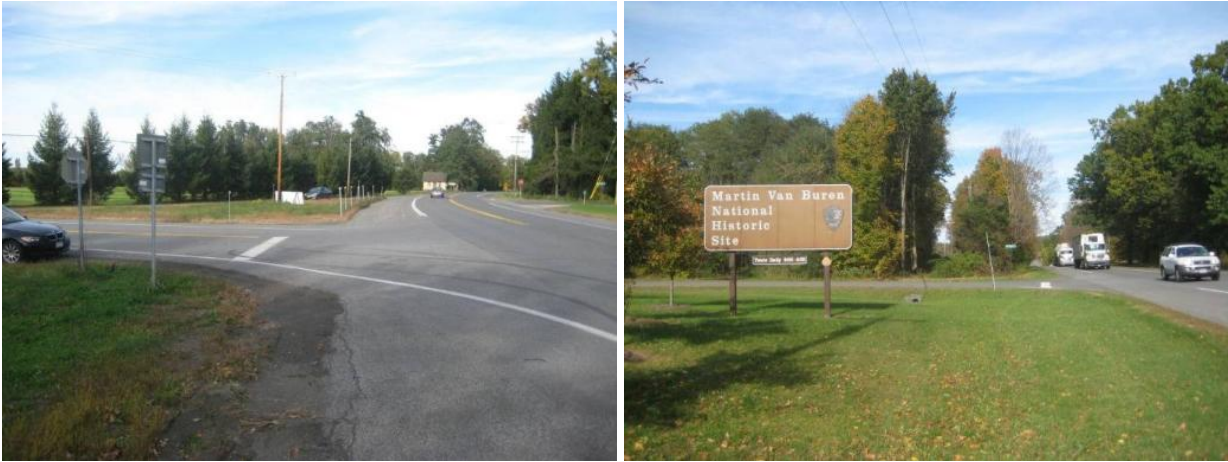
Figure 8 Looking north at SR 9H and County Road 21 junction (left), looking north from the park entrance (right) Source: Volpe Center
