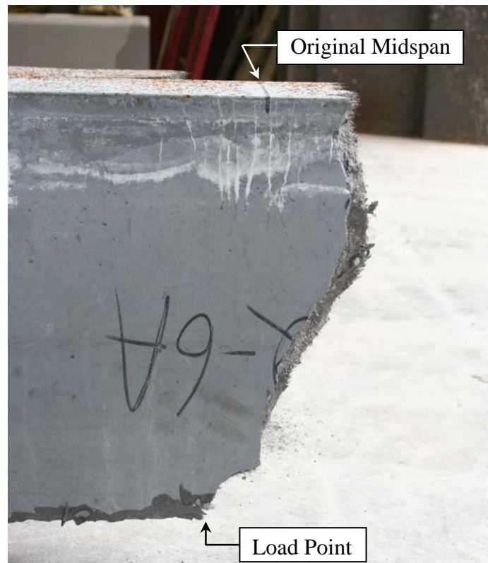
Figure 24. Photo. Elevation view of failure location.
