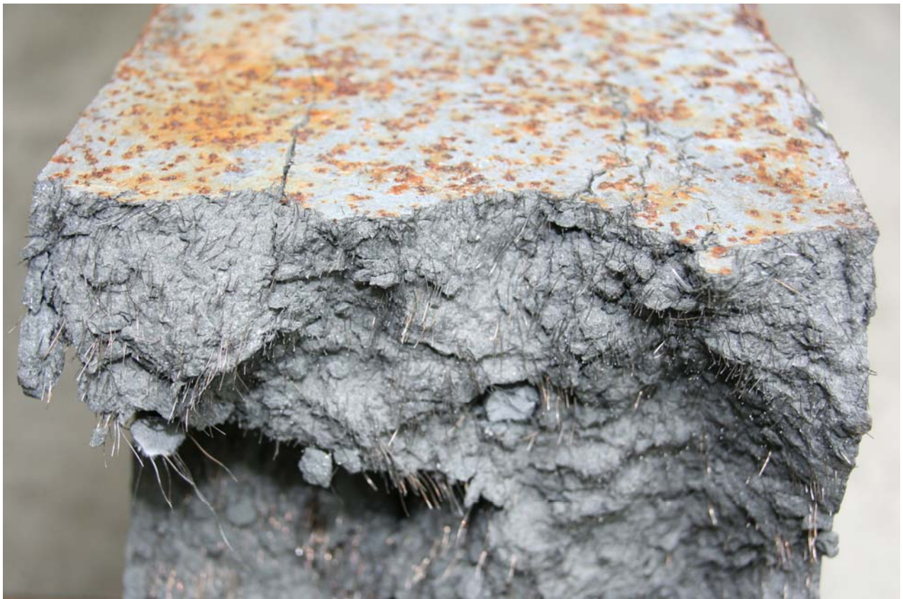
Figure 26. Photo. Close-up of failure surface.
