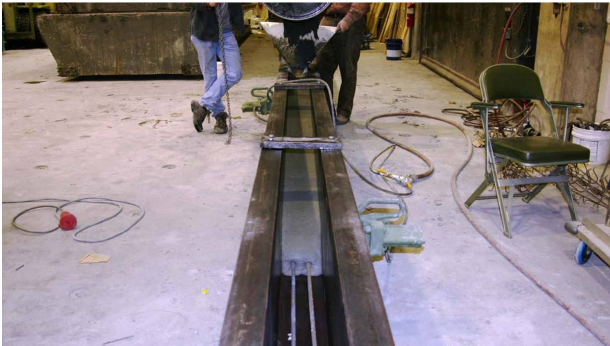
Figure 2. Photo. Placement of UHPC into beam form.
