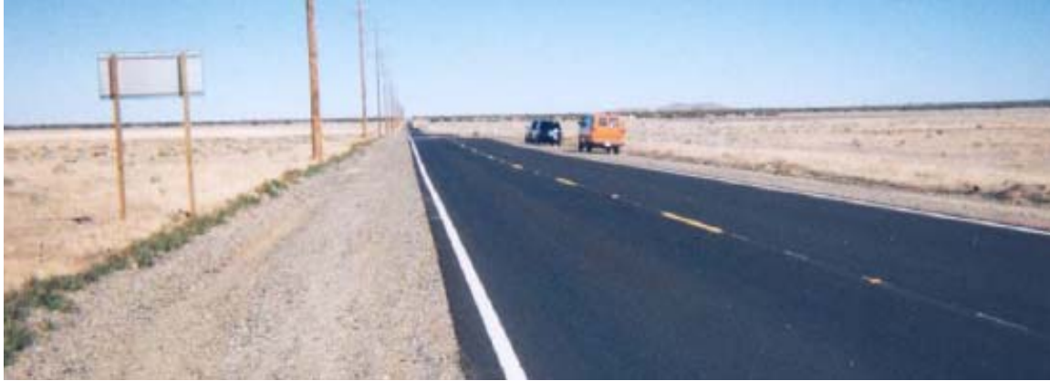
Figure 2. LA138 pavement testing area photograph.
