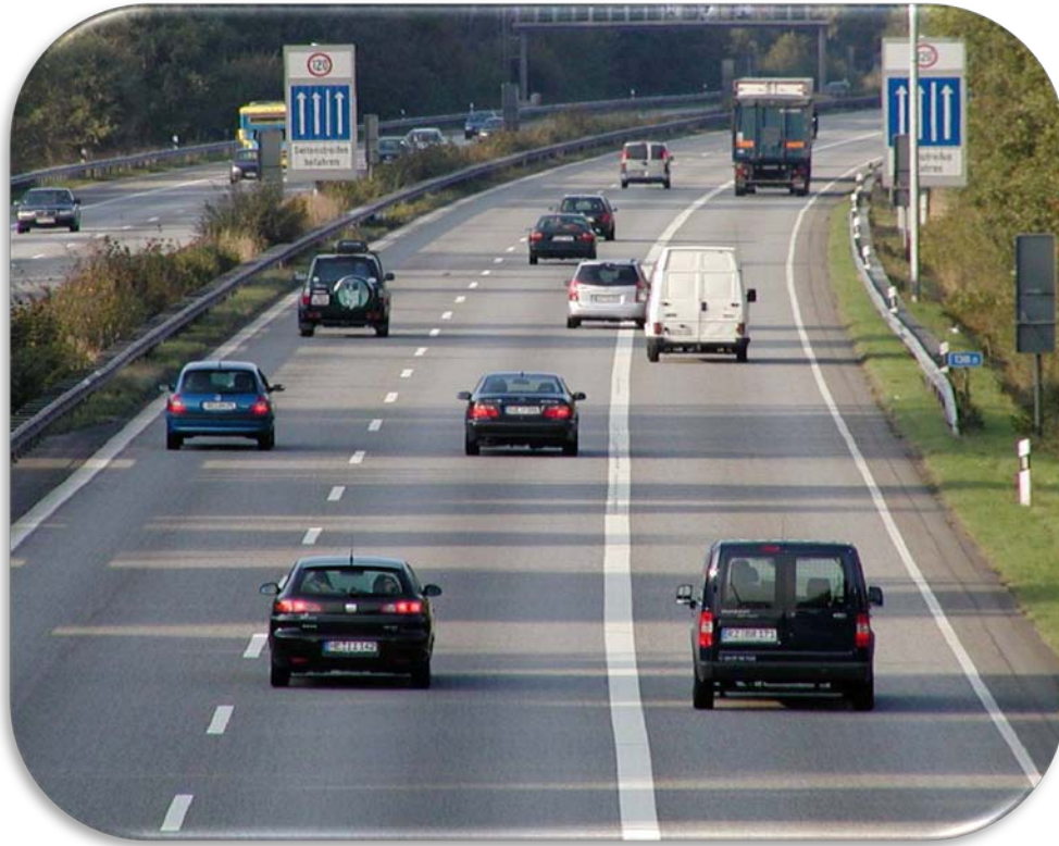
Figure 5. Photo. Temporary Shoulder Use—Germany (13) .
