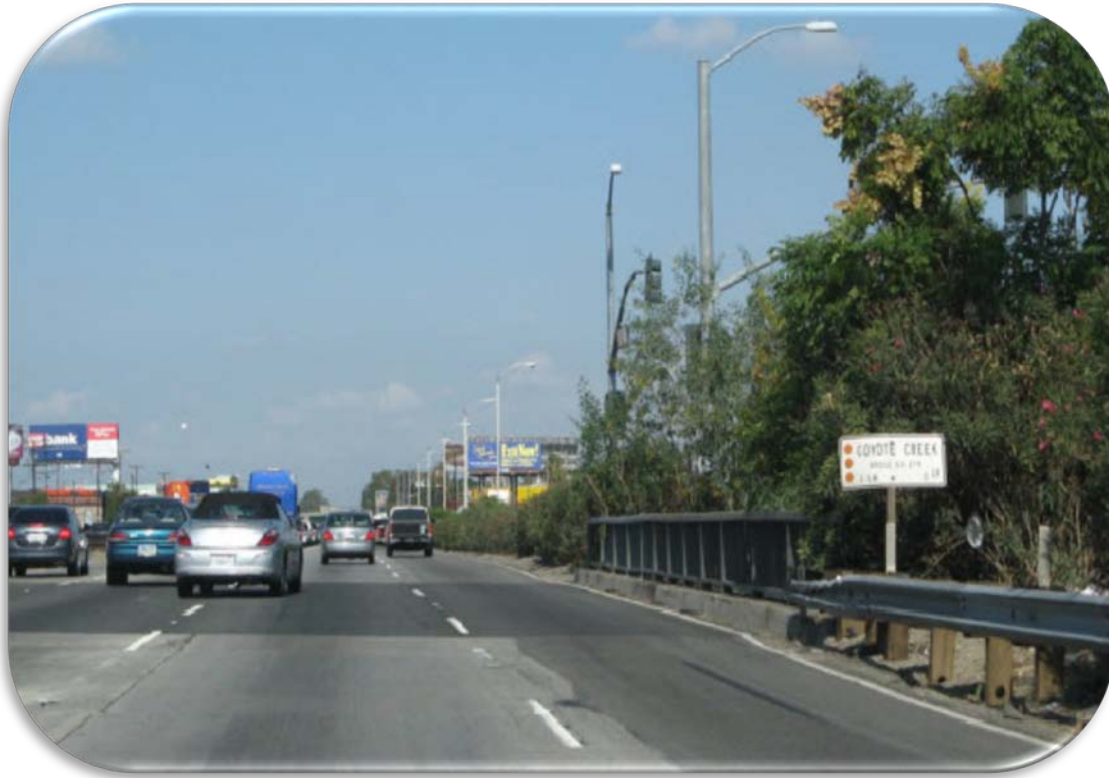
Figure 10. Photo. Converted Shoulders on I-5—California (Photo Courtesy of CALTRANS).
