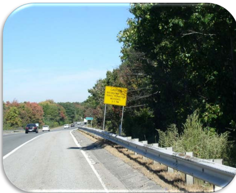
Figure 22. Photo. Warning Shoulder Use Sign (Photo Courtesy of MassDOT). (23)
