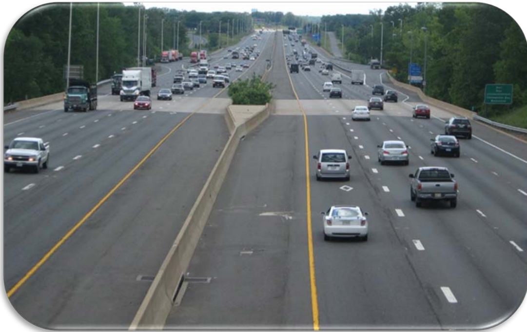
Figure 40. Photo. I-66 HOV Lanes, West of HOV/SL Portion—Virginia (50) .
