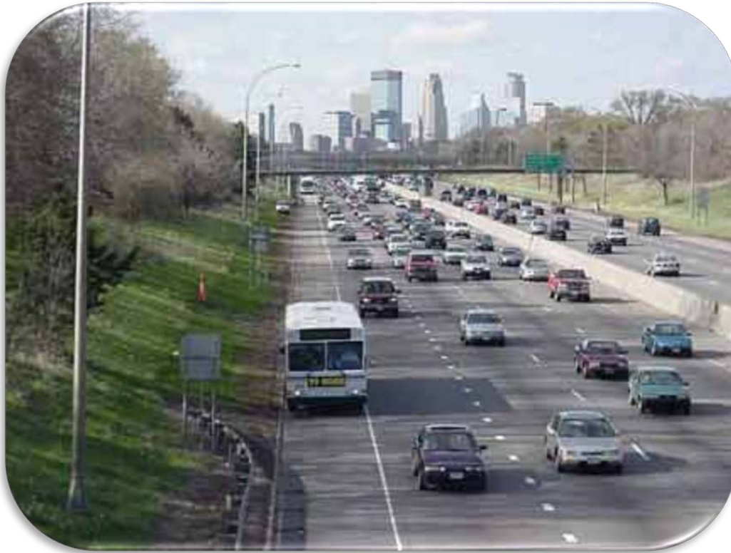
Figure 9. Photo. Bus on Shoulders—Mn/DOT (Photo courtesy of Mn/DOT).
