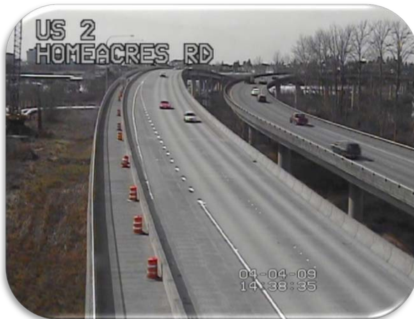
Figure 47. Photo. US 2 Shoulder Use—Everett, Washington. (55)
