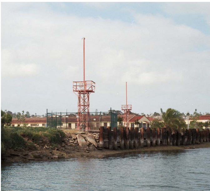
Figure 1-5 SAN MALSR Land-based Platforms
