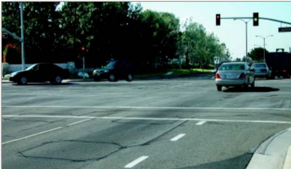
FIGURE 4 Loop detectors, signified by the black wires embedded in the pavement at the intersection below, are a common type of traffic counting device
