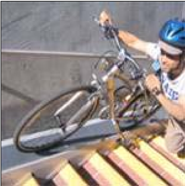
Figure 45 - Bicycle stair channel
