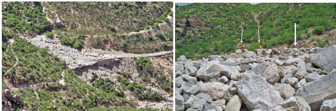
Figure 21 – Aerial (left) and ground (right) photos of debris flow deposits burying the end of the tram road in Sabino Canyon. The tram road turnaround is beneath the boulder pile in the ground view; note Lee Allison and Todd Shipman of the AZGS for scale. Large white arrow points to the location of buried rest room facilities. Aerial photo provided by R.H. Webb. 32
