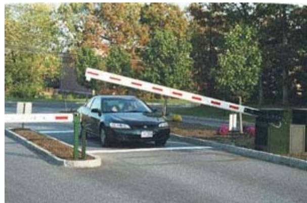
Figure 42 - Automatic vehicle access control 103
