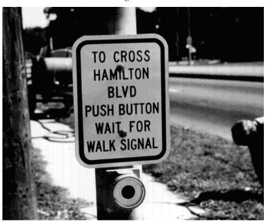
Figure 3-21. Manually operated pedestrian push button.
