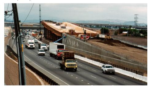
Figure 1-2. Freeway-to-freeway HOV bypass lane structure under construction at intersection of CA–57 and CA–91 freeways in Anaheim, CA (Photograph courtesy of Lawrence A. Klein).
