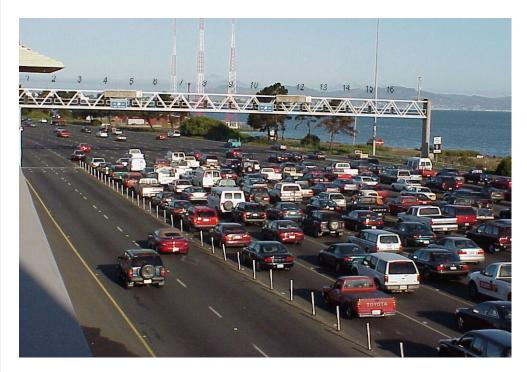
Figure 3-12. Mainline metering configuration on I–80 westbound crossing the San Francisco-Oakland Bay Bridge (Photograph courtesy of Caltrans District 4, Oakland, CA).
