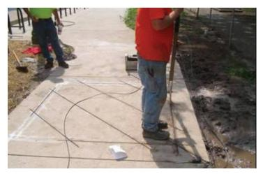
Figure 4-29. Type D loop installation (Photograph courtesy Darcy Bullock, School of Civil Engineering, Purdue University, West Lafayette, IN).
