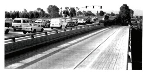
Figure 3-13. Freeway mainline metering at El Cajon, CA.
