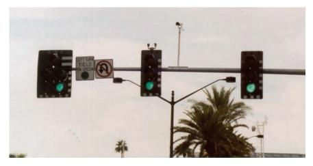
Figure 1-6. Overhead camera mounting on a mast arm as typically used to provide imagery to a VIP for arterial signal control (Photograph courtesy of Lawrence A. Klein).
