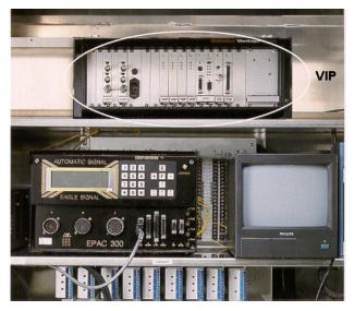
Figure 2-51. Video image processor installed in a roadside cabinet (Photograph courtesy of Iteris, Anaheim, CA).
