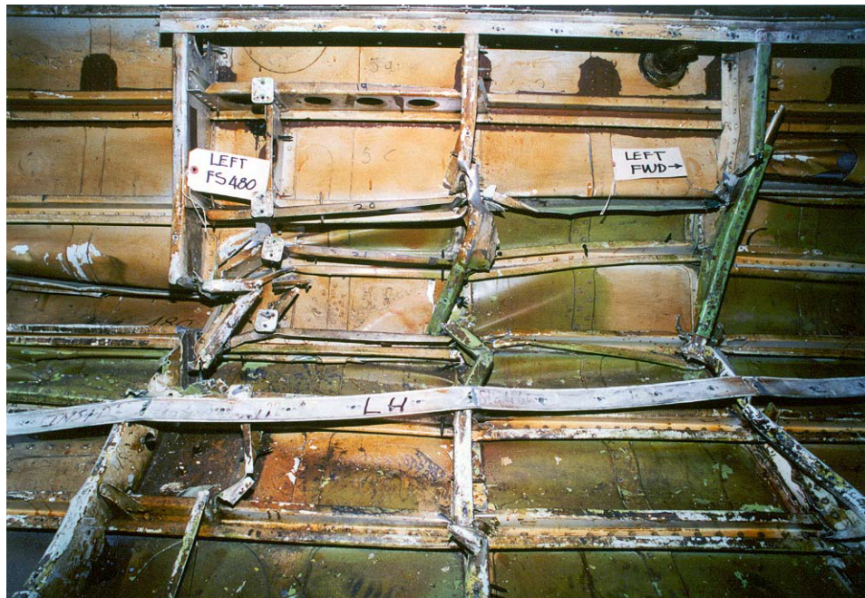
FIGURE C-76. CARGO AREA—LEFT SIDE CLOSE-UP
