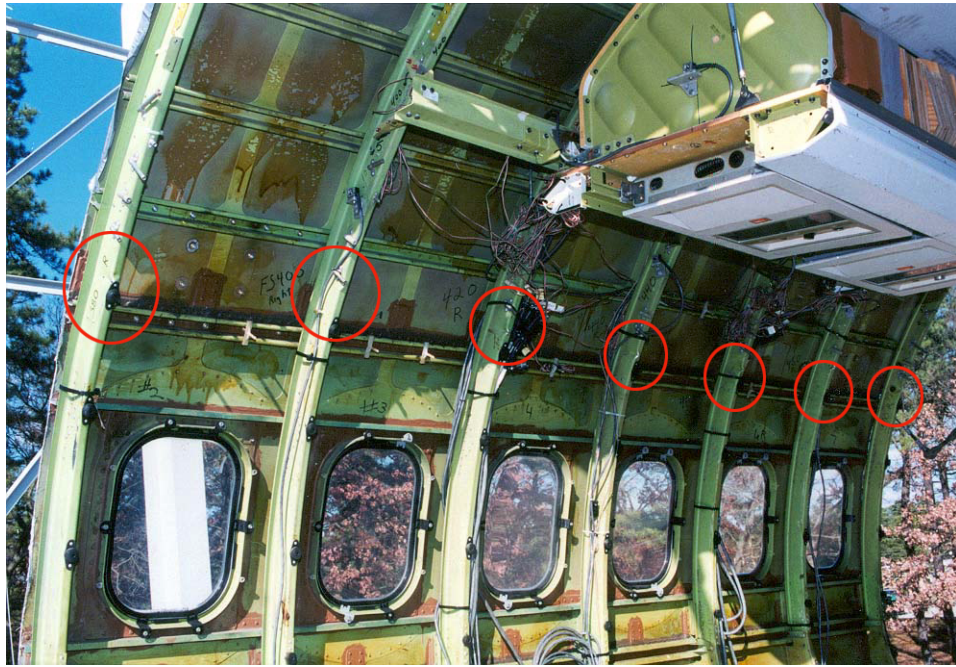
FIGURE C-63. CRACKED FRAME SECTIONS—RIGHT SIDE
