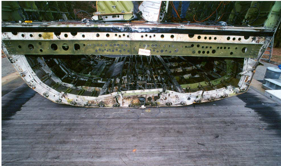
FIGURE 52. FRONT VIEW—FRACTURED CARGO FRAMES
