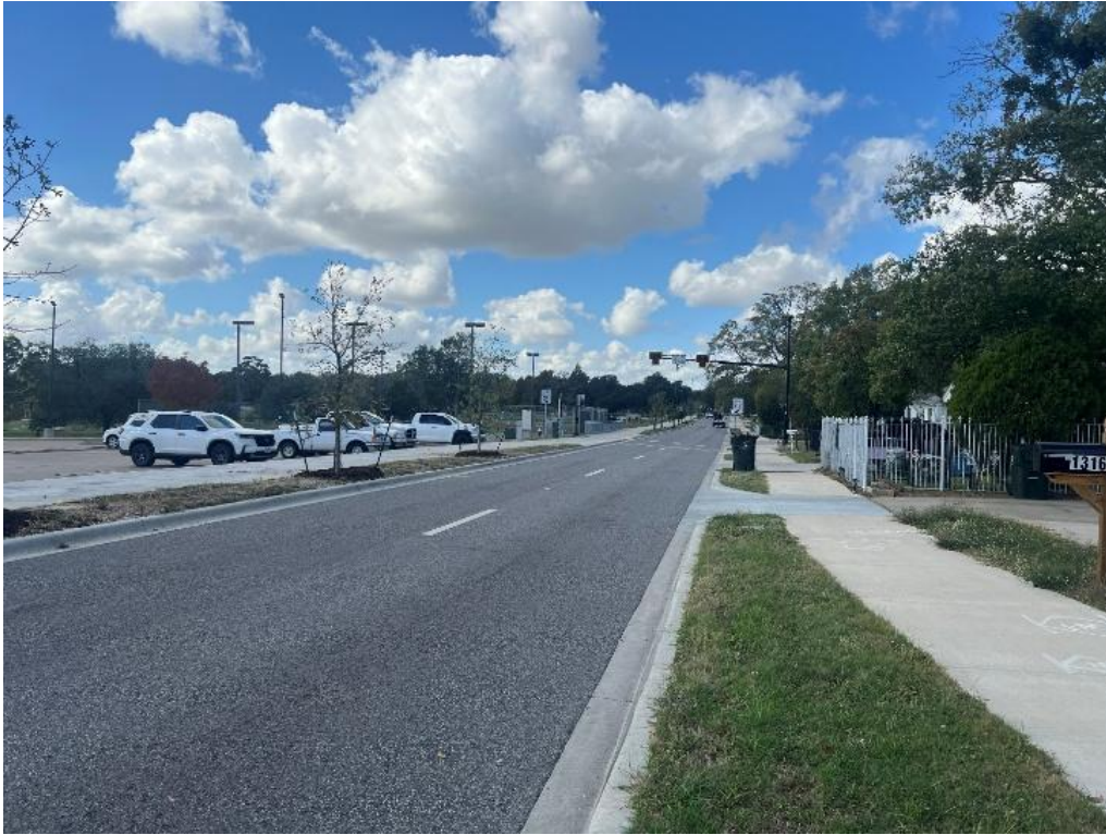
Figure 13. Cross Section for FM 158 after Construction; Pedestrian Hybrid Beacon Added at Cross Street Along with Wider Sidewalks and Reallocation of Shoulder.
