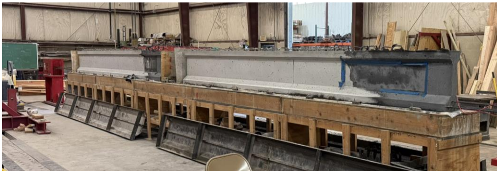
Figure 17. Completed hybrid specimen showing intermixing of SCC and UHPC
