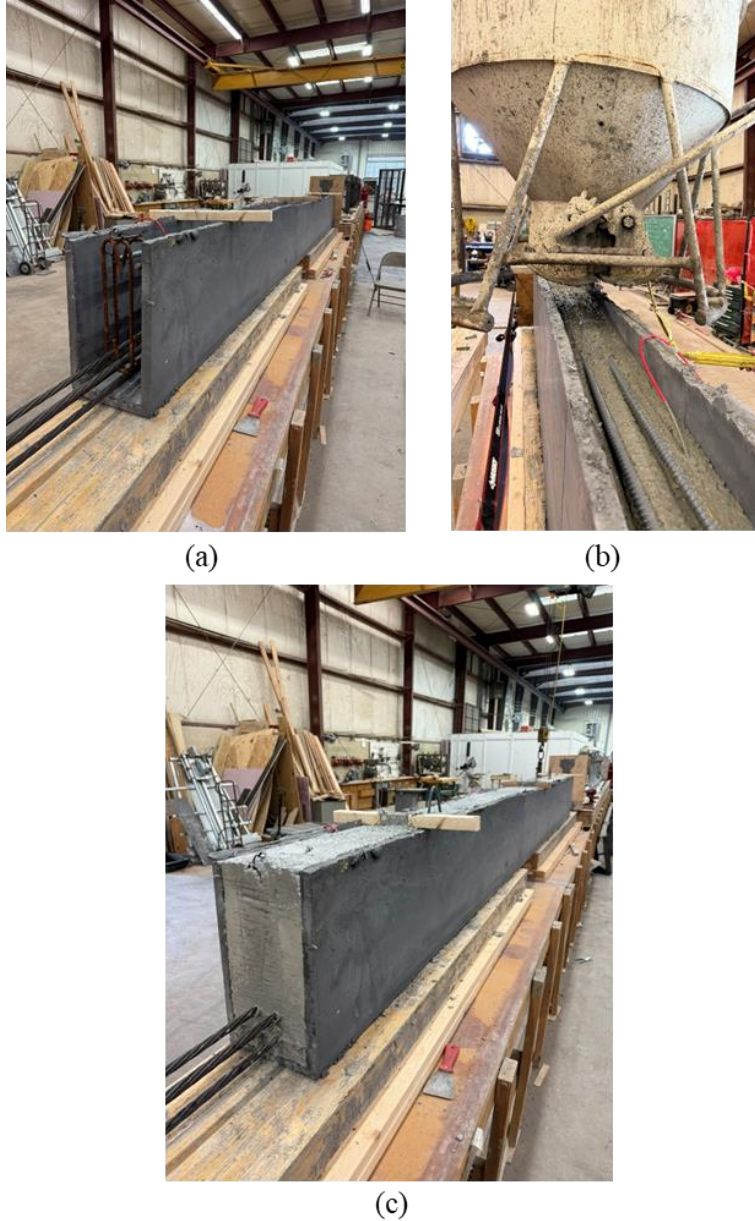
Figure 25. UHPC shell prestressed girder (a) before casting, (b) during casting, and (c) after completion
