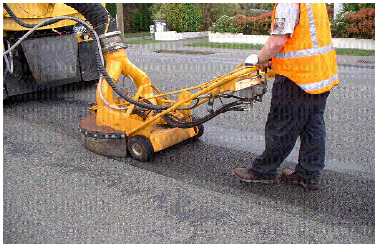
Figure 20. UHP Water Cutting.
