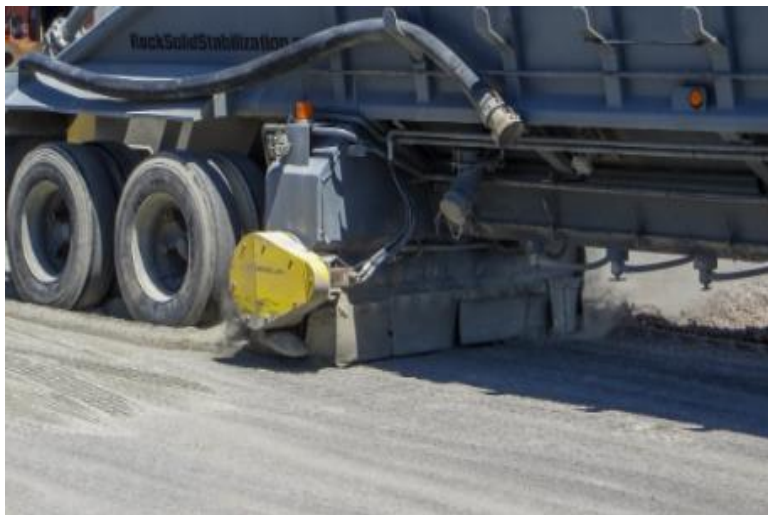
Figure 19. Cement Stabilized Base.
