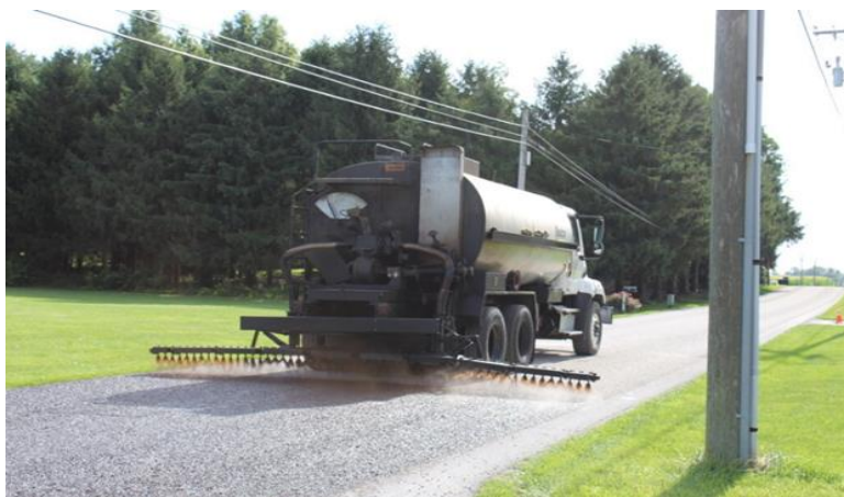
Figure 10. Fog Seal.
