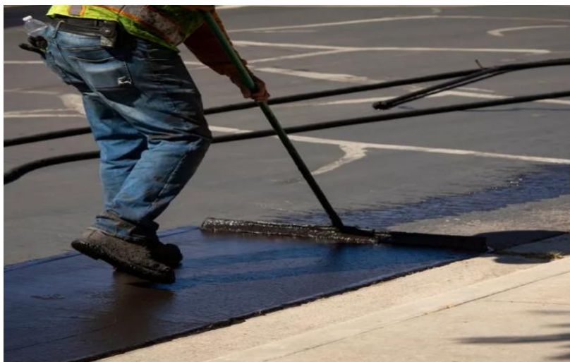
Figure 16. Spot Seal.
