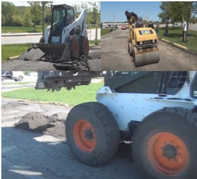
Figure 15. Base Repair.
