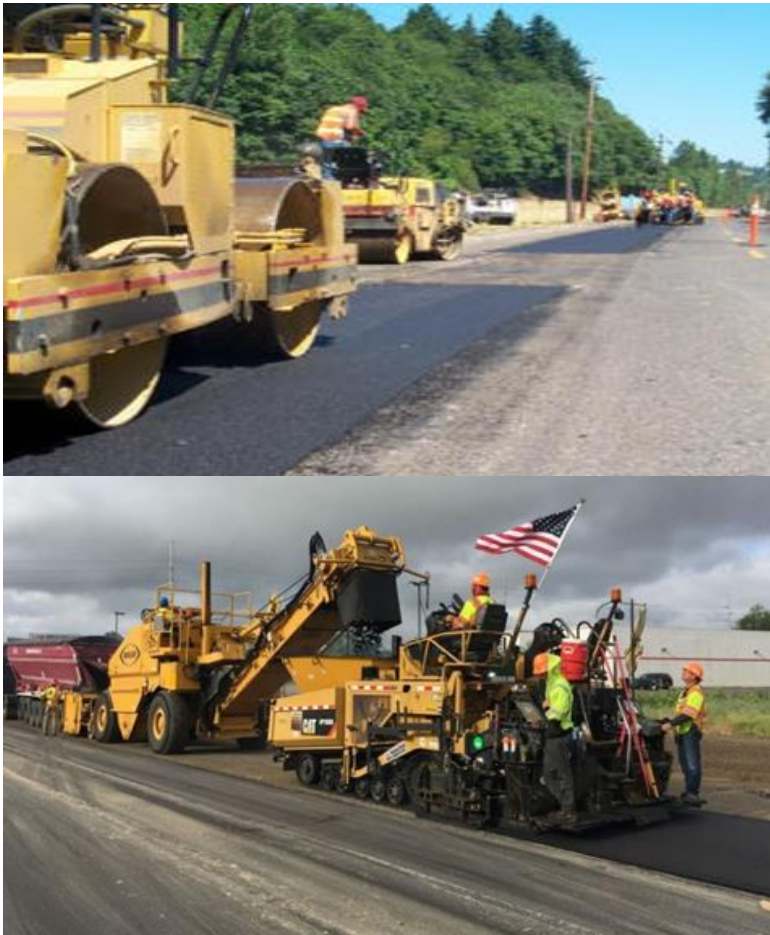
Figure 13. Level Up and Overlay.
