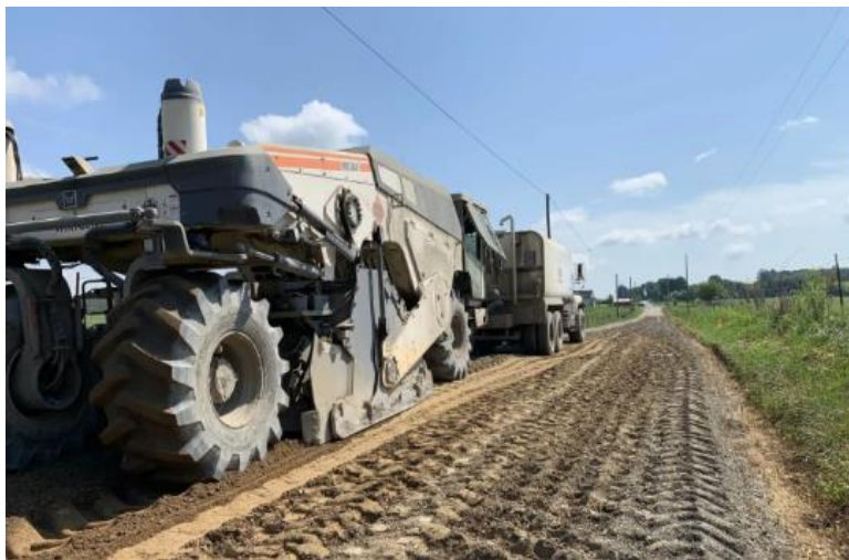
Figure 18. Full-Depth Reclamation.
