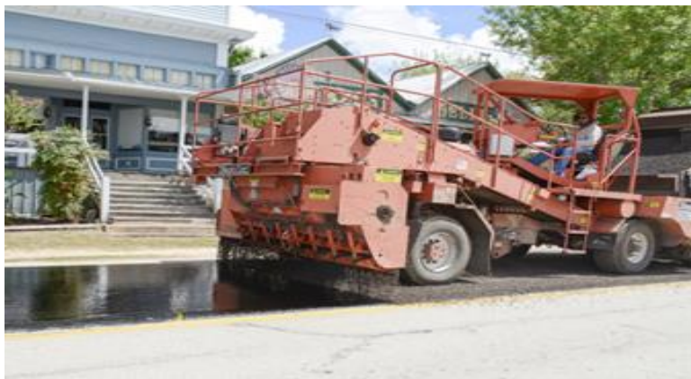
Figure 11. Seal Coat.
