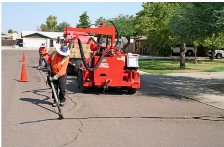
Figure 9. Crack Seal.
