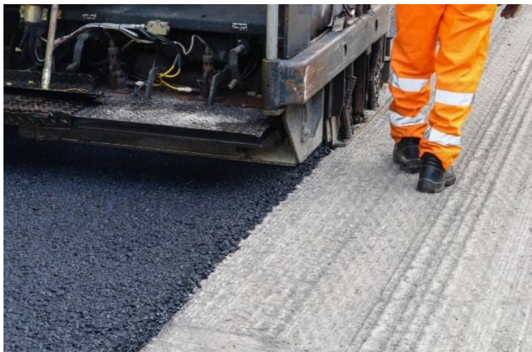
Figure 14. Mill and Overlay.
