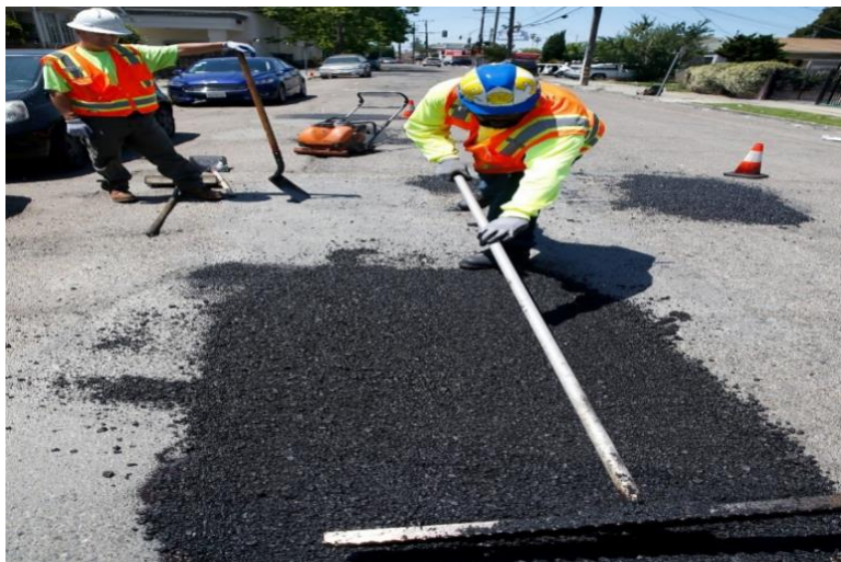
Figure 21. Pothole Repair.
