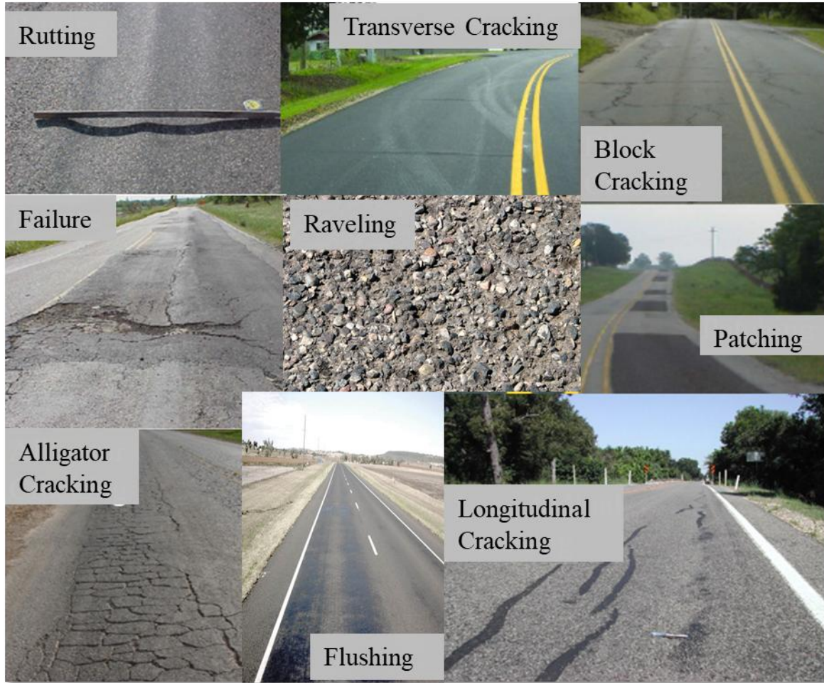
Figure 4. Flexible Pavement Distresses.
