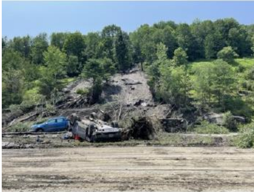
Figure 6.4 July 11, 2023, debris flow at Route 62, Railroad Street, Barre, VT. (Credit: VTrans)
