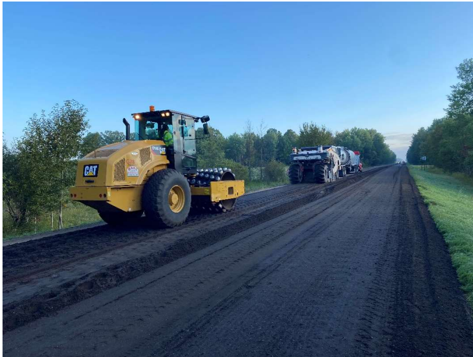
Figure 5: Initial compaction of FDR using Sheep-foot or Pad-foot Roller.
