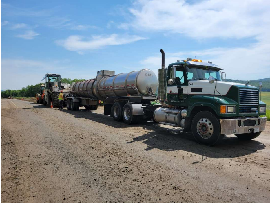
Figure 4: Reclamation pass of VTrans Marshfield-Danville project in 2024.
