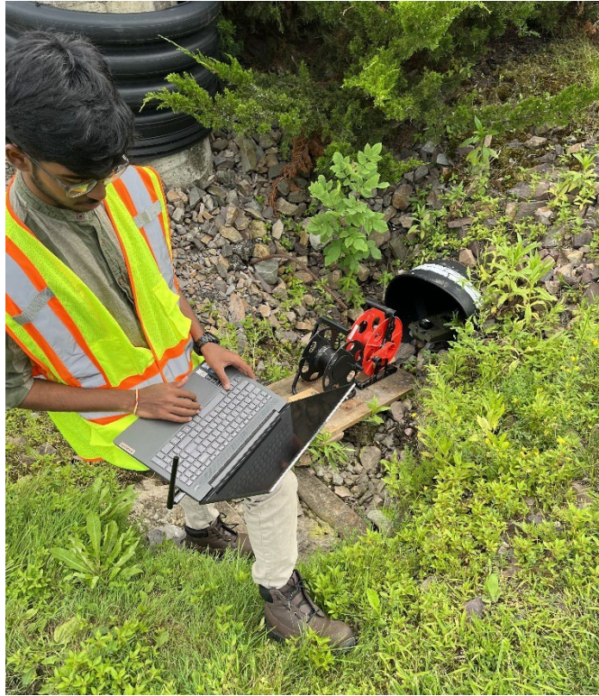
Figure 7 18-inch corrugated plastic culvert inspection setup
