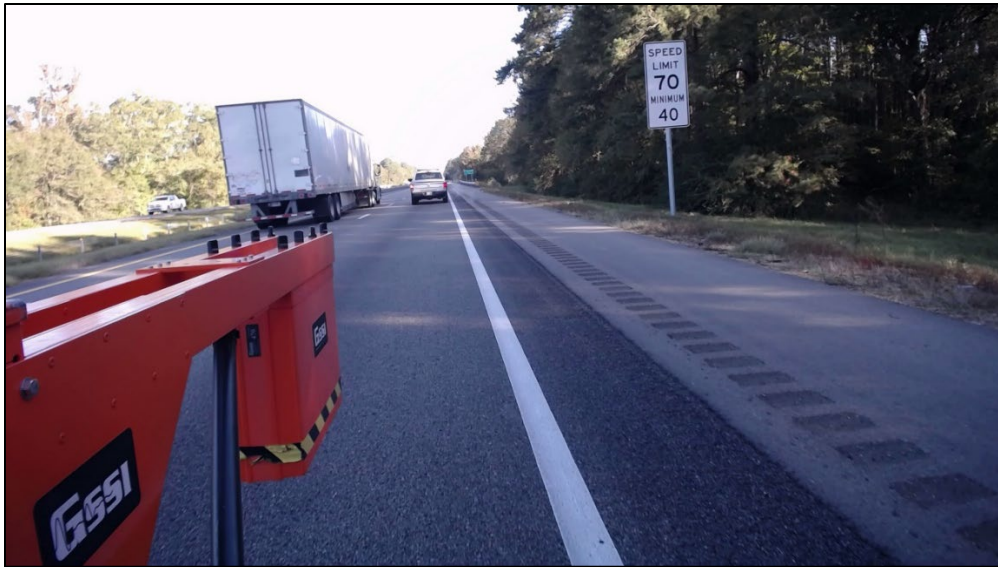
Figure 10. Example ROW Image at Station 52+75 NB
