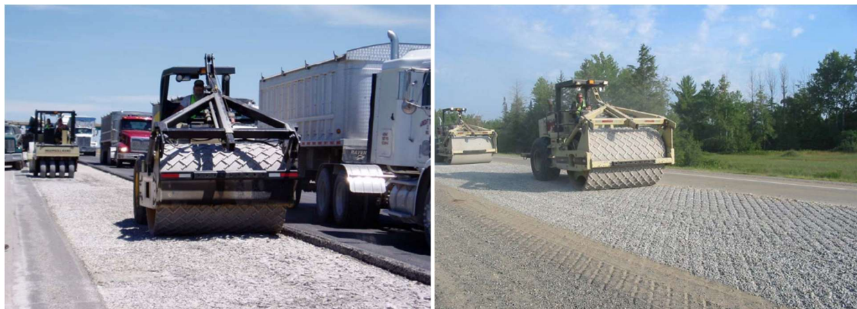
Figure 7. Frequently the Z-grid roller is followed by a steel-wheeled or pneumatic tire roller (29, 30) .
