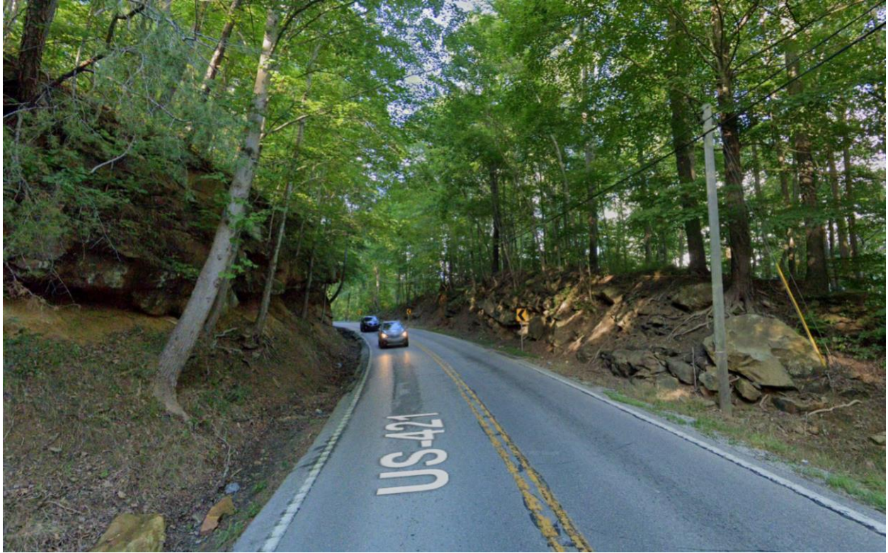
Figure 6.8 US 421 Curve, No Shoulder, Limited Visibility, Trees Fall Across Roadway
