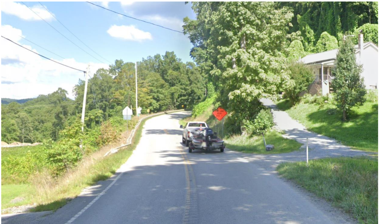
Figure 6.5 US 421 Steep Grade, Unsigned, Poor Visibility
