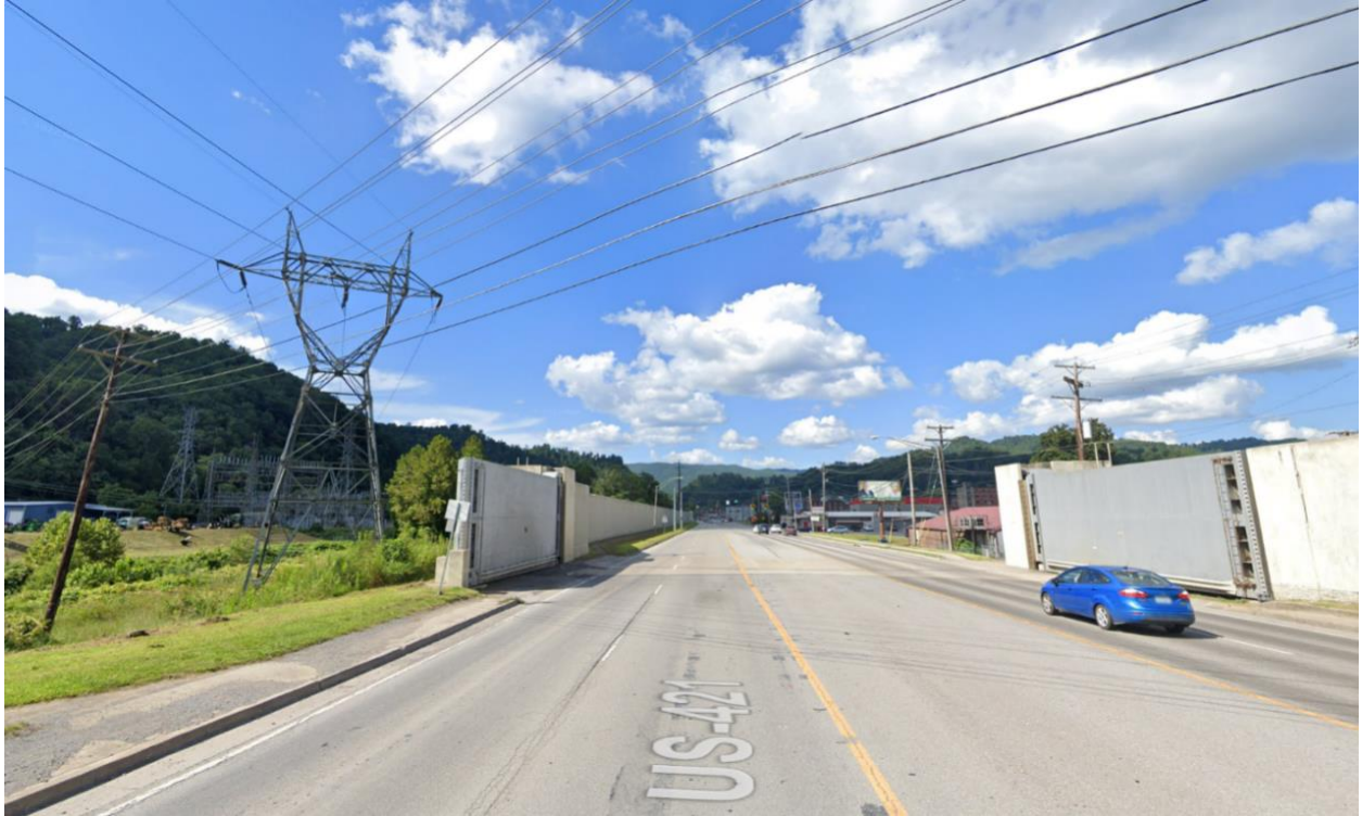
Figure 6.14 US 421 Flood Wall in Harlan
