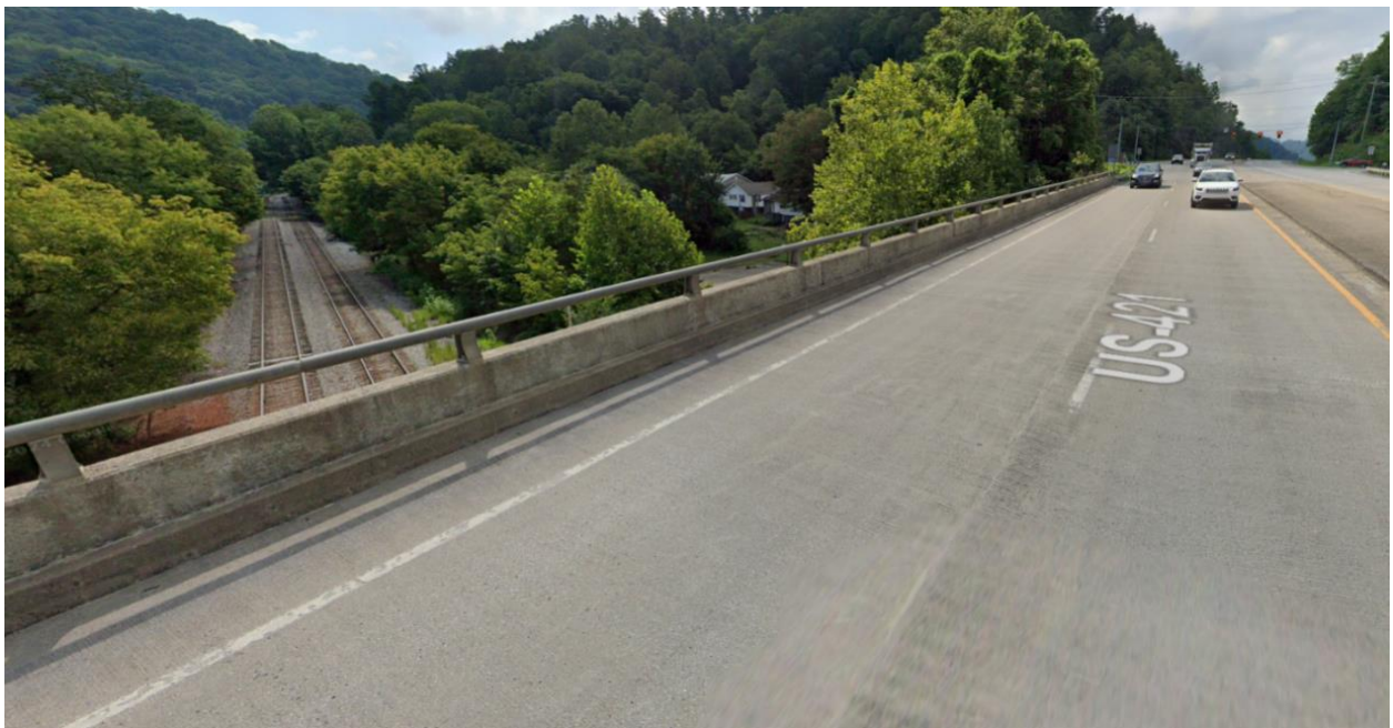
Figure 6.13 US 421 Bridge Crossing Railroad
