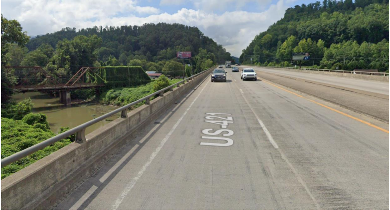
Figure 6.12 US 421 Bridge Crossing Water
