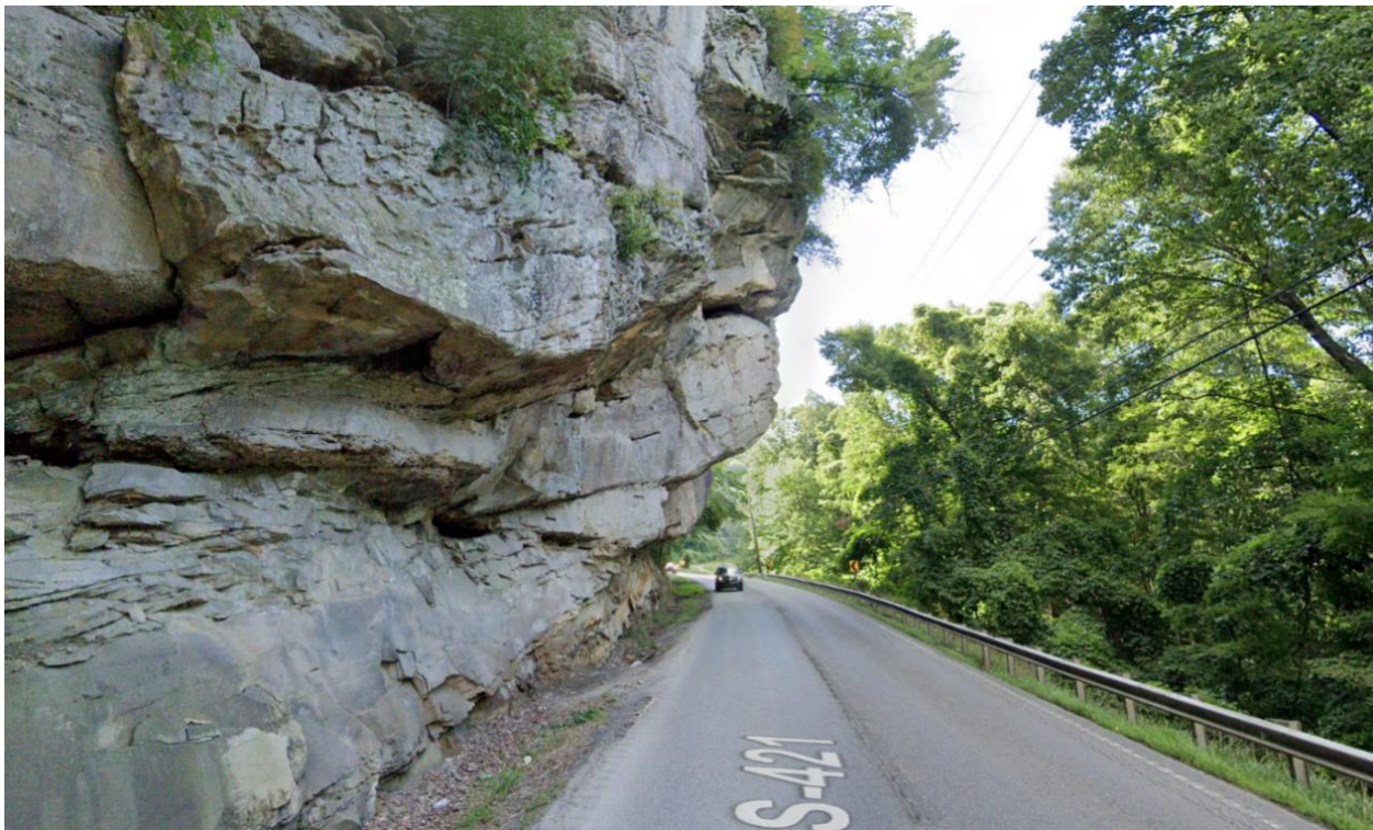
Figure 6.7 US 421 Mountains, No Shoulder
