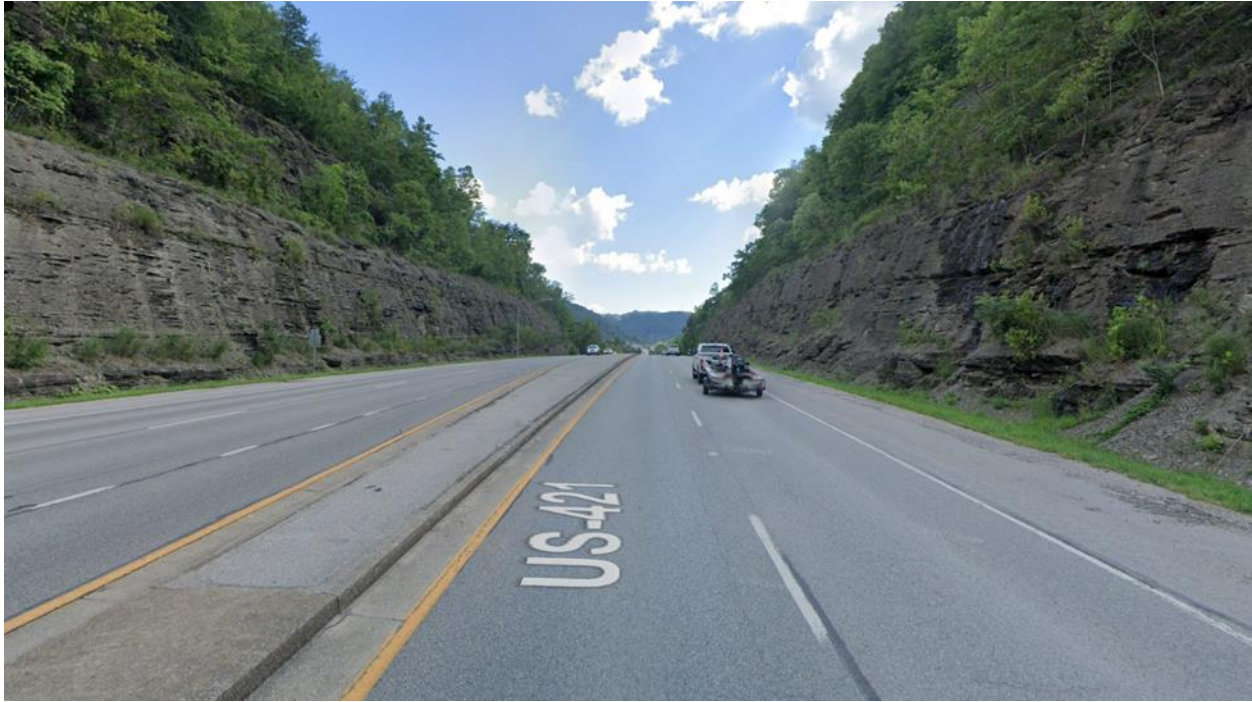
Figure 6.10 US 421 Wider Right of Way and Shoulders, Cut Through Mountain
