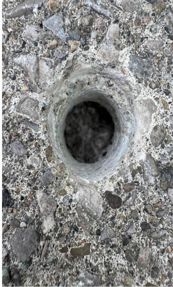
Figure 3.11 Sampling Hole After Collection of Concrete Deck Dust
