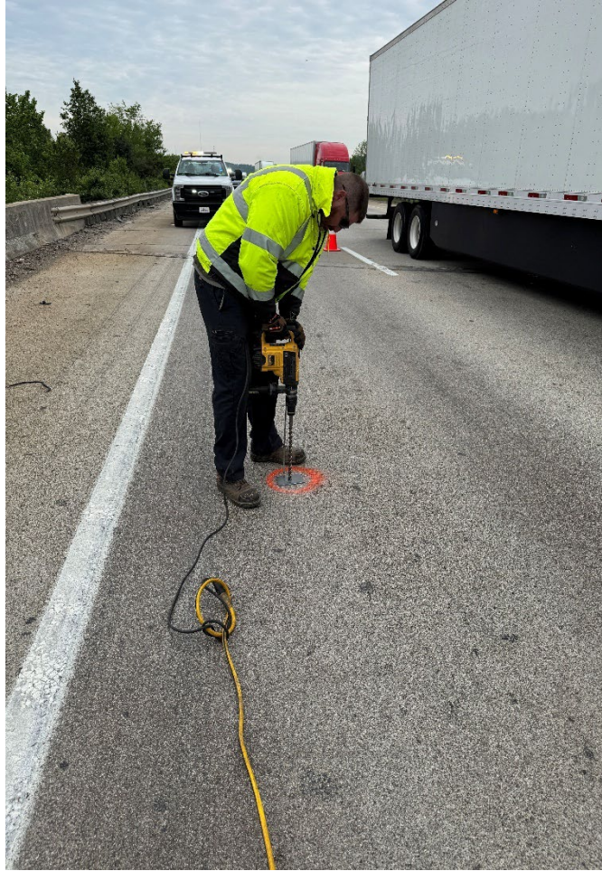
Figure 3.10 Drilling for Chloride Sample in the Wheel Path
