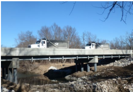
Bridge Live Load Testing
