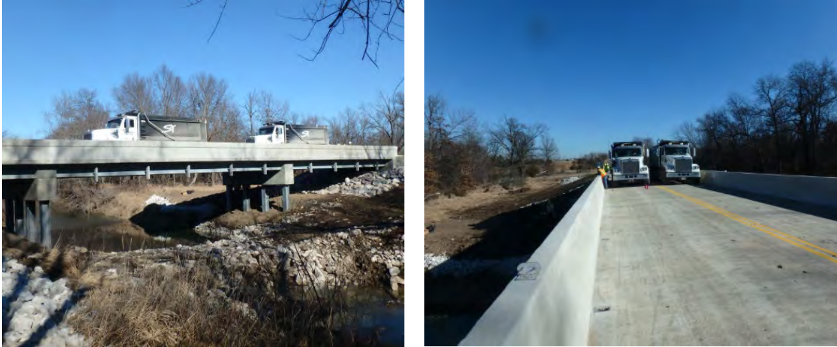
Figure 3-17. Truck loading during live load testing.
