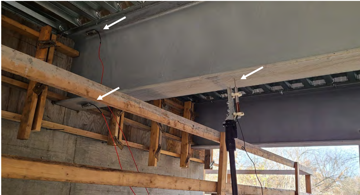
Figure 3-8. Picture of ST and LVDT placement for dead load testing.
