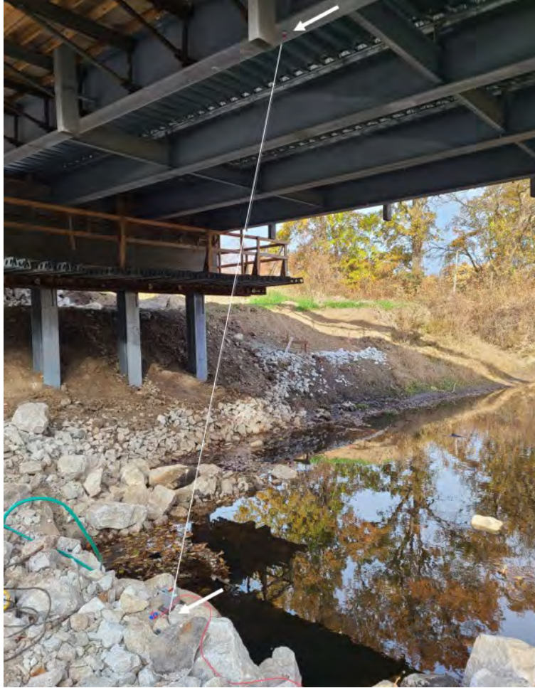
Figure 3-9. String pot placement at midspan for dead load testing.
