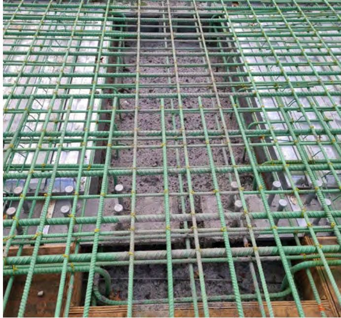
Figure 3-4. Concrete diaphragm at bent no. 3 before the concrete deck pour.
