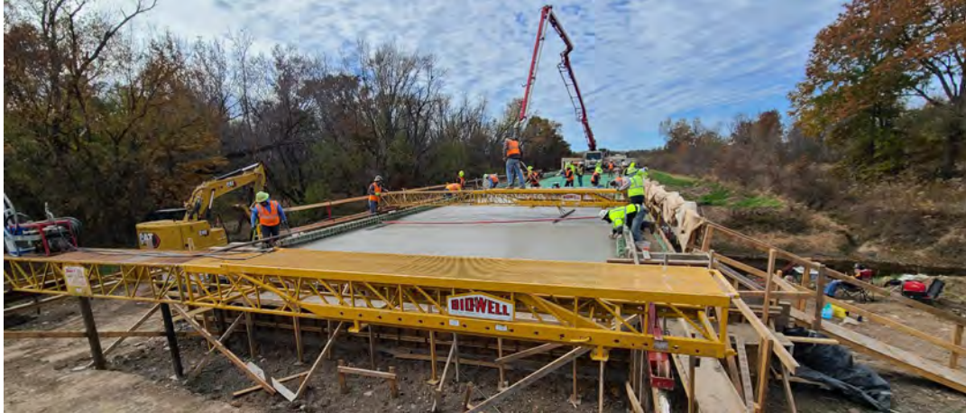
Figure 3-10 Deck pour starting at bent 4.
