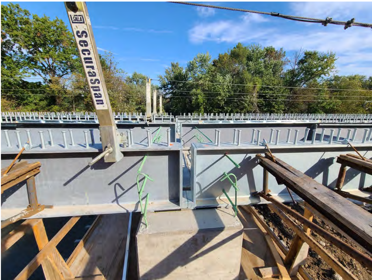
Figure 3-3 Steel girders on bent cap before first diaphragm pour.
