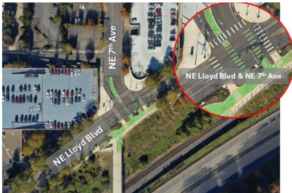
Figure 4-3. Location and intersection layout of the rest-in-red installation at NE 7th Avenue and NE Lloyd Boulevard in Portland, Oregon
