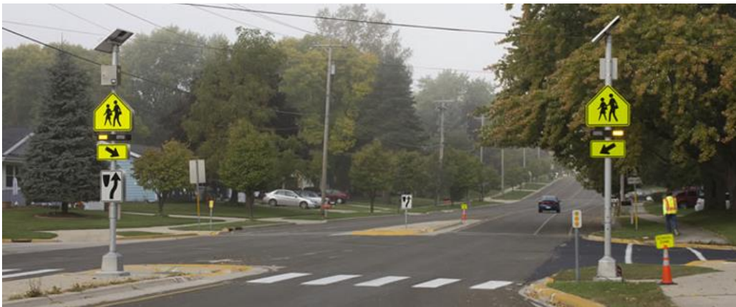
Figure 3-2. Rectangular rapid flashing beacon
