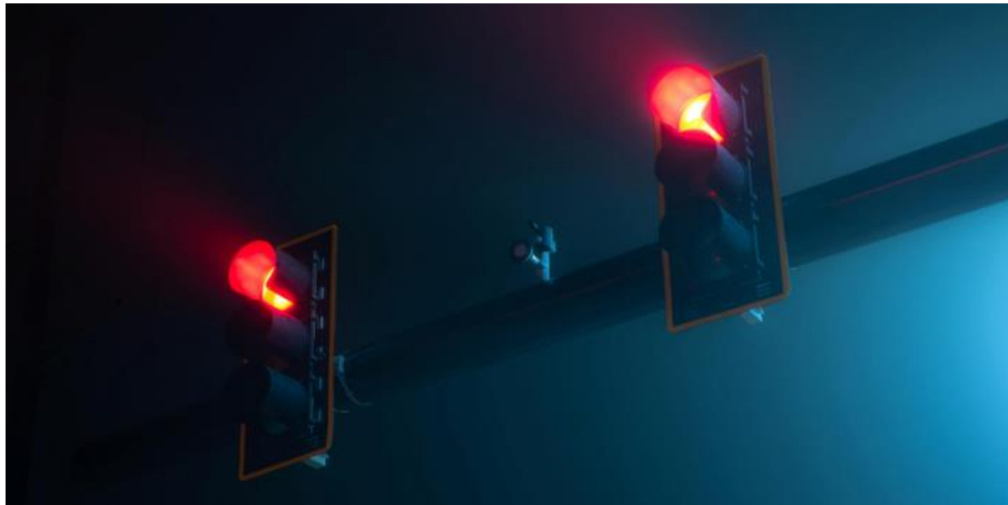
Figure 2-9. Example of rest-in-red signal display during nighttime operation
