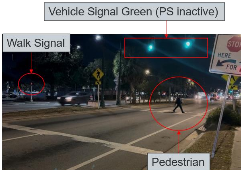
Figure 5-16. Example of a noncompliant pedestrian crossing at the Fletcher Avenue PS at midblock site
