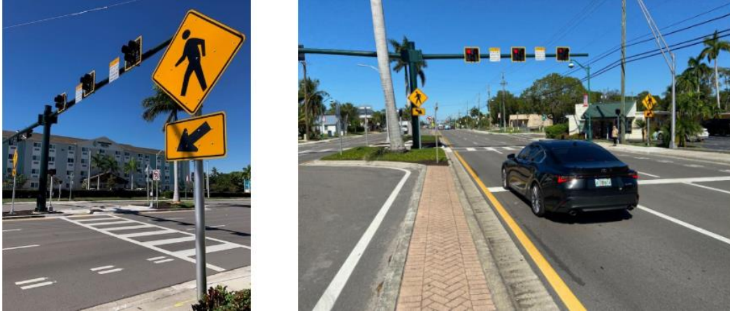
Figure 2-6. Midblock PHB installed on US-41 in Lee County, FL (FDOT / Lee County Outreach, 2024)
