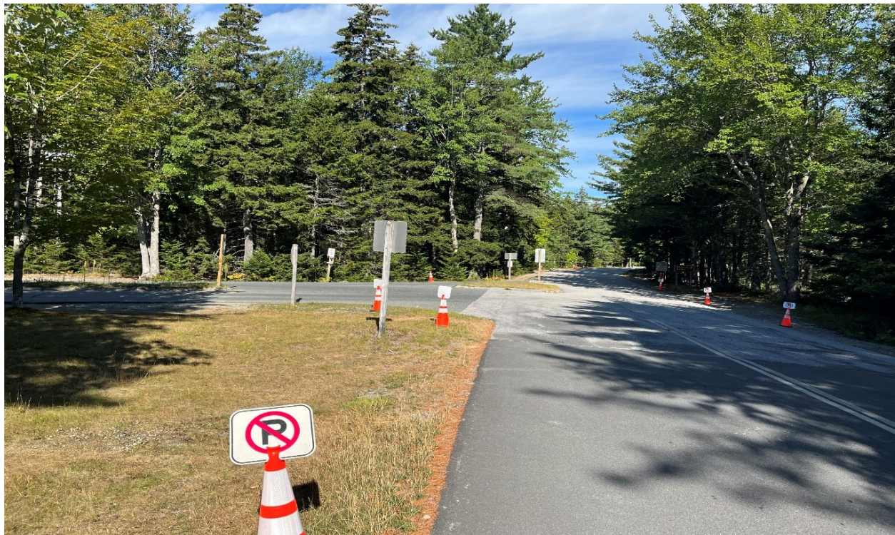
Figure 17: Traffic Cones and Temporary Signage around Confusion Corner
