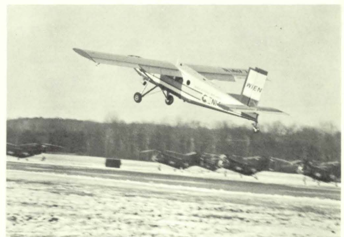
EIGHT-place, Swiss-built Pilatus Turboporter, first single-engine turboprop aircraft to win an FAA type certificate. Easy to handle, its short takeoff and landing characteristics make it exceptionally useful for bush operations in Alaska.
