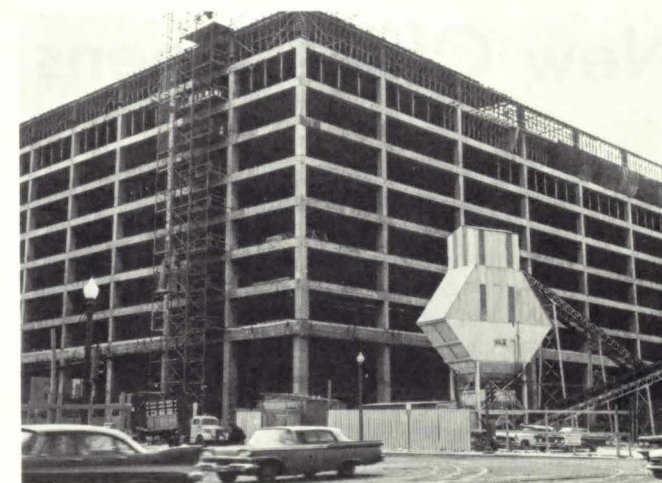
FOB 10, the Agency's future home on Independence Ave., near the Smithsonian Institute in Washington, begins to take shape. The 10-story, ultra-modern office complex is scheduled for occupancy by Agency personnel in 1963.
