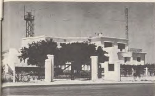
REGIONAL ATCC at Tunis, Tunisia, has typical architectural lines of country.
