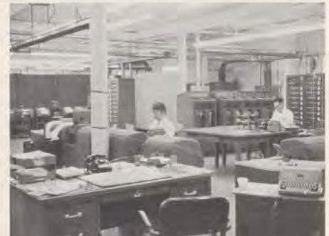
THE ADIS in Kansas City's Telecommunications Center; (center) Service "B" teletypewriter loop; (right) "A" and "C" teletypewriter loop in background with automatic relay units at right center and portion of "B" loop in foreground.
