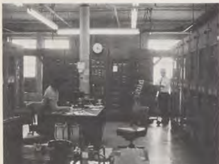
THE ADIS in Kansas City's Telecommunications Center; (center) Service "B" teletypewriter loop; (right) "A" and "C" teletypewriter loop in background with automatic relay units at right center and portion of "B" loop in foreground.
