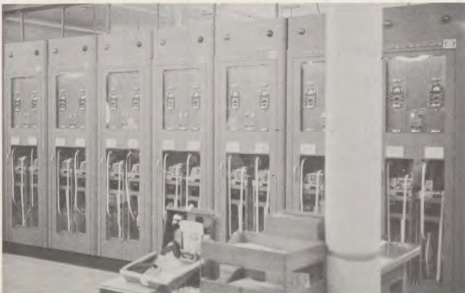
HIGH to low speed converter circuits; (right) 800 WPM high speed reperforators and 100 WPM transmitter-distributor.
