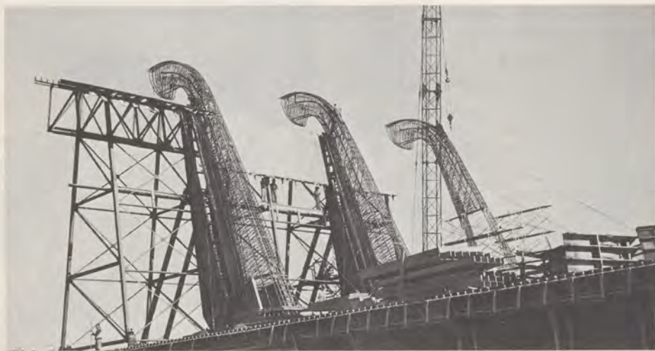
FRAMEWORK for three of the sixteen 65-foot concrete pillars for Dulles International Airport's modernistic terminal roof is shown being installed.
