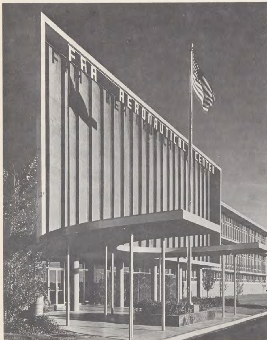
FACADE OF FAA Aeronautical Center Administration Building at Oklahoma City.
