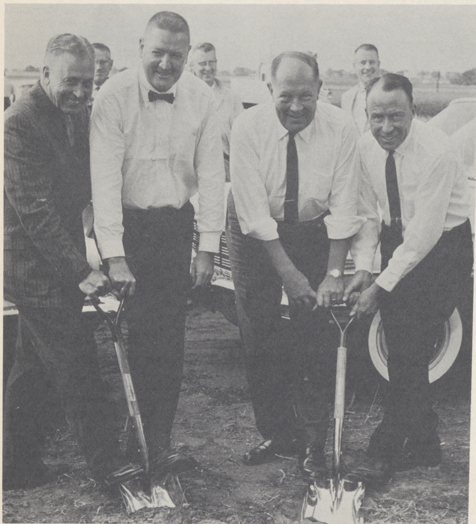
GOLDEN shovels glisten as ground is broken for new Denver Air Traffic Control Center Building at Longmont, Colo. From left, L. M. Wilkins, general contractor, Lt. Governor Robert Knous, Walter P. Plett, Region 4 Manager and Albert Will, Mayor of Longmont.
