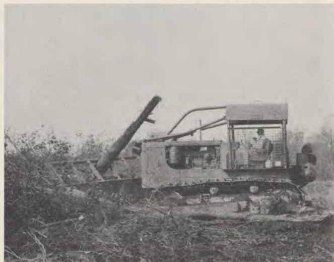
Before any construction could begin at Dulles, more than 12 million cubic yards of earth had to be excavated; more than 300 structures removed or demolished. Huge cats devoured the hedgerows and bowled over trees which were in the way. Hummocks were leveled, valleys filled, immense trenches opened and closed again over thousands of feet of pipes and conduits.
