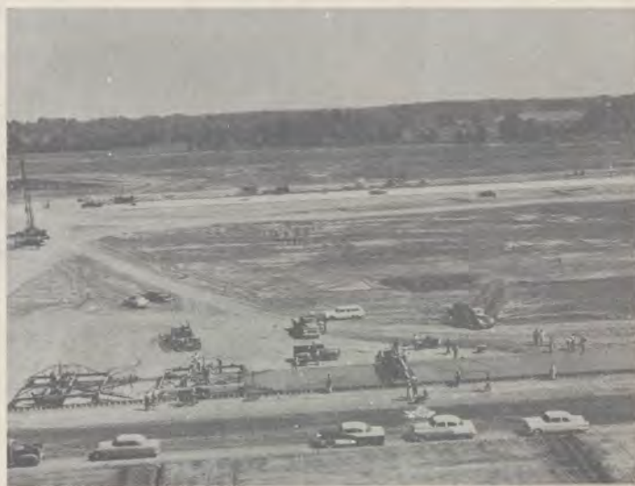
Aerial view of two parallel North-South runways which are 11,500 feet long and 150 feet wide and the 10,000 foot long and 150 foot wide Northwest-Southeast runway. Paving work called for laying about 1,196,000 square yards of Portland cement concrete.
