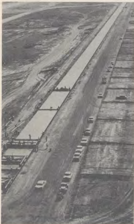
One 25-foot wide strip of concrete almost reaches the end of one 11,500 foot runway.
