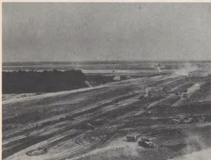
Before any construction could begin at Dulles, more than 12 million cubic yards of earth had to be excavated; more than 300 structures removed or demolished. Huge cats devoured the hedgerows and bowled over trees which were in the way. Hummocks were leveled, valleys filled, immense trenches opened and closed again over thousands of feet of pipes and conduits.
