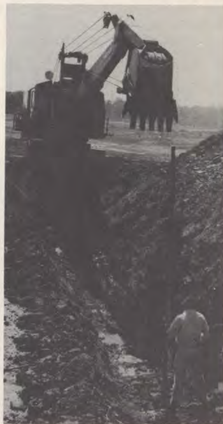
Steam shovel scoops out debris after blasting has taken place to make room for drain pipes and electrical conduits.
