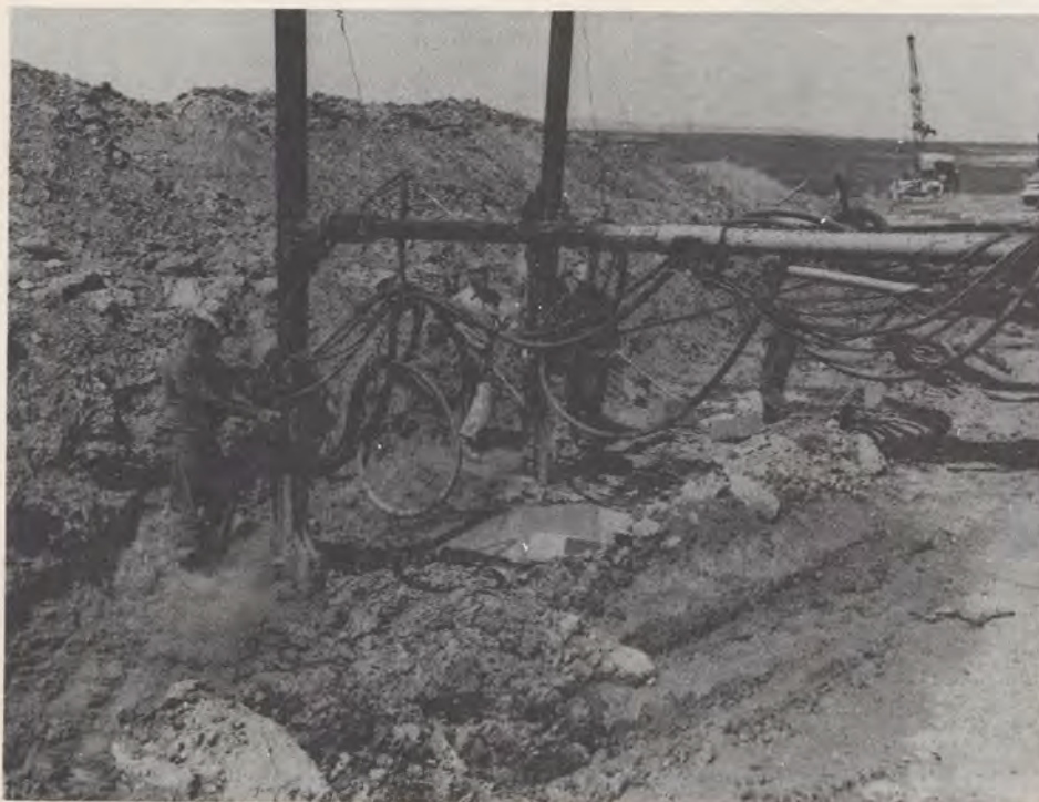
Construction workers use multiple pneumatic drill in preparatory work before blasting to make room for drainage ditch. Drills were also used for foundation exploration work.
