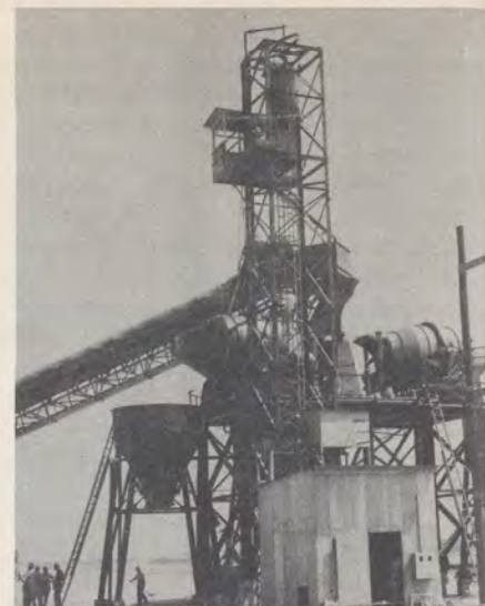
Close-up of one part of the cement plant showing ramp which fed the plant and chutes which dropped cement into waiting trucks.
