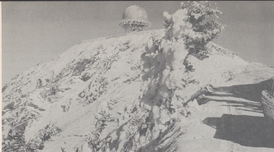
Long range radar on mountain top in Wasatch range overlooks Salt Lake City. It's powerful antenna spots aircraft within a radius of 200 miles and up to 60,000 feet.
