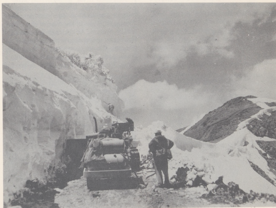
During construction on roadway to Francis Peak long-range radar site, workers plow through 60-foot snow drift in the middle of summer to reach men on the other side.
