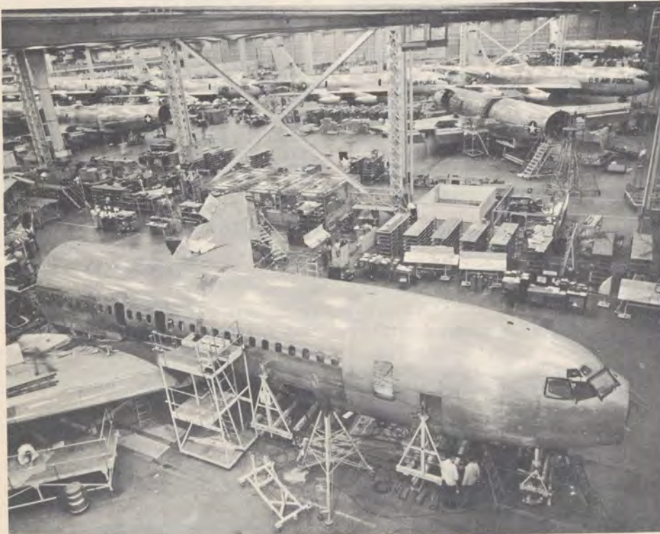
Another view of the Renton production line. In the foreground and second row, wings are being joined to the bodies of 707s. Manufacturing inspectors will check the operations.
