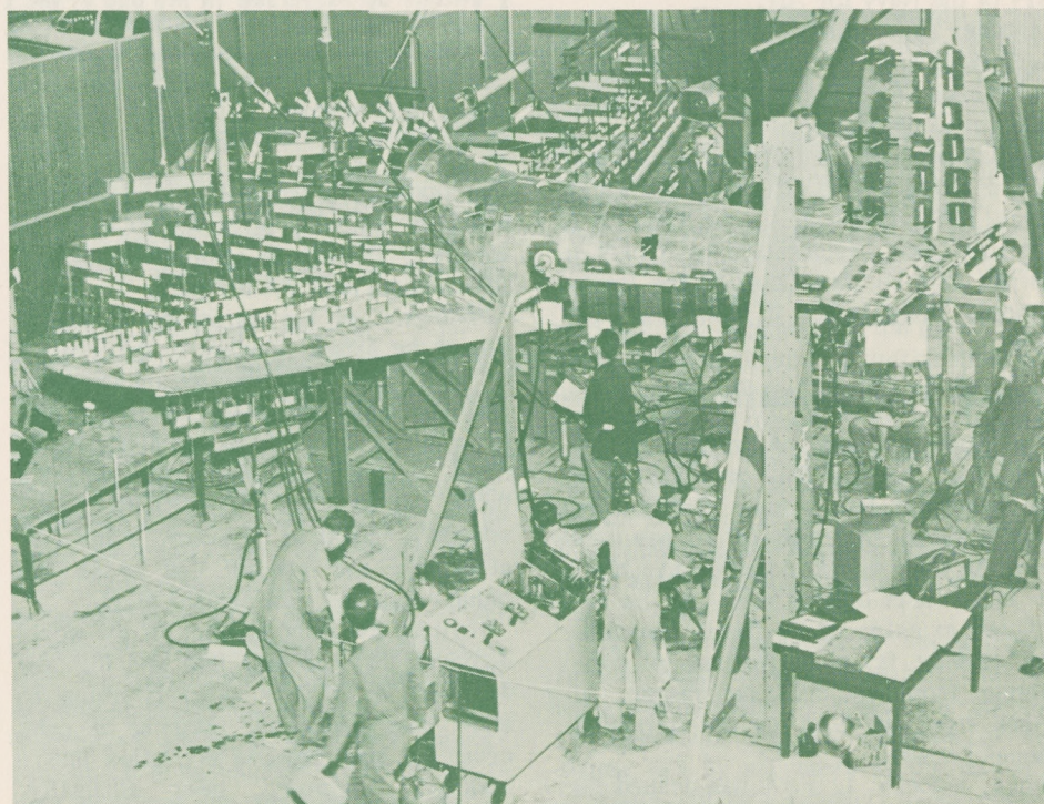
A typical static test setup in a structural testing area shows test loads being applied with hydraulic jacks through a whiffle tree system to tension pads located on the test specimen.
