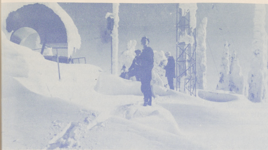
Rime ice is a problem and drifts get high around RCAG building on Big Mountain.
