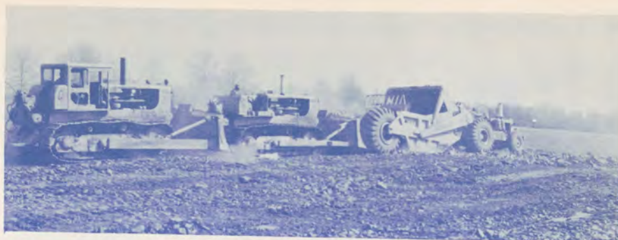
Grading underway at Chantilly
