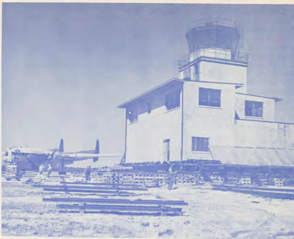
ATLANTIC CITY: This strange traffic situation developed on runway 8-26 at the National Aviation Facilities Experimental Center in Atlantic City, where a five-story control tower is being moved half a mile to a new location. Workman at extreme left signals C-119 that all is clear while 1,300-ton structure inches forward on its perilous passage across the field. Engineers estimate journey will be completed in 12 days. When settled on its new foundation, tower will overlook dual 12,000-foot parallel runways to be constructed at Bureau of Research and Development's field facility.
