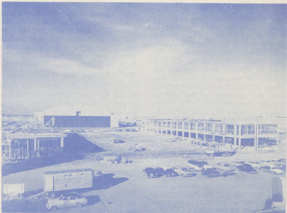
New Hangar 9 is being erected on the empty ground in the center of the picture. The lean-to additions are shown being erected on the east and west sides of the hangar. These lean-to's will furnish office and laboratory space.
