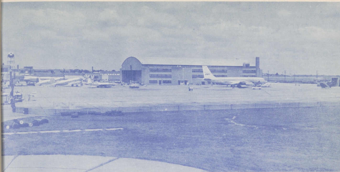
Exterior view of new Hangar 8 at the Aeronautical Center, built for FAA by the Oklahoma City Airport Trust. The hangar measures 180 feet by 280 feet. A Boeing 707 jet is shown parked alongside.
