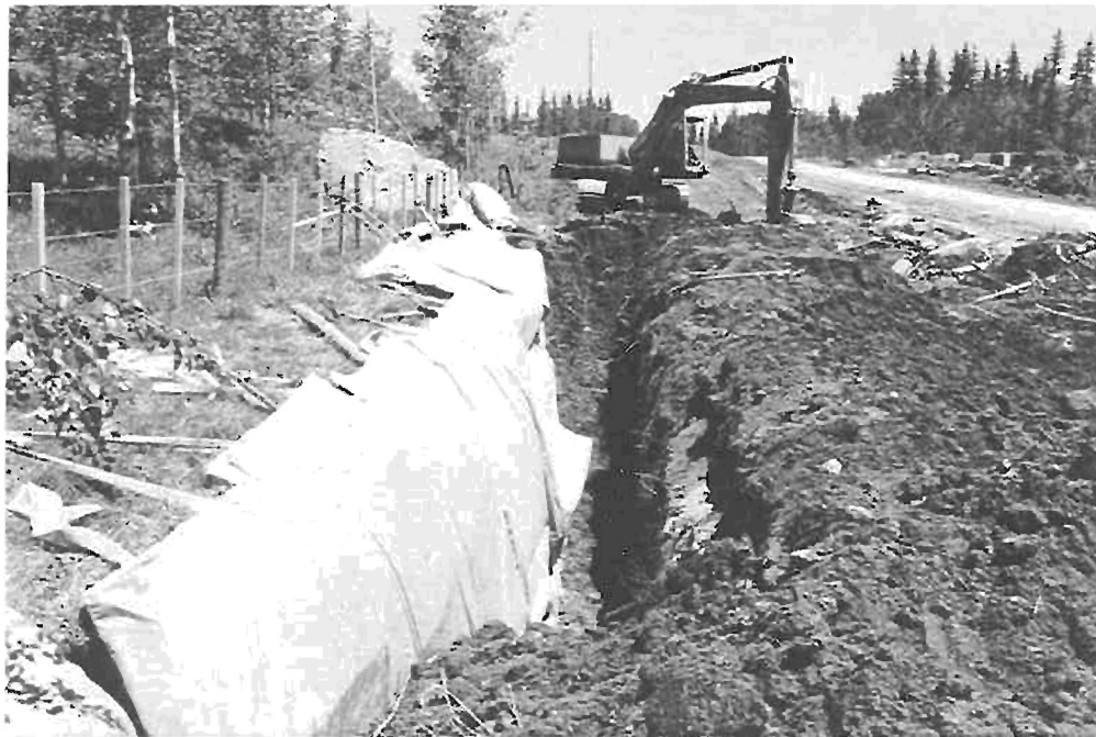
Figure 4 Pictured here is the installation on the south end of the project. The trench was dug in relatively dry soil which made it easy to hang the curtain drain sections from the fence, place them neatly and backfill the trench.
