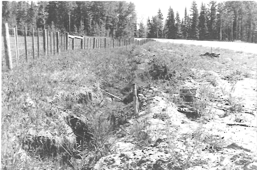
Figure 15 This moisture tube is adjacent to the interceptor ditch on the uphill side of the curtain drain.
