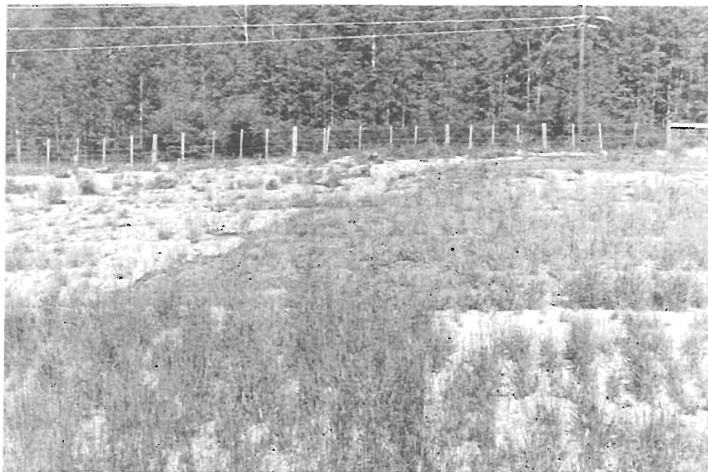
Figure 10 The dark area in the middle of the photo is where the surface is saturated on the slope below the interceptor ditch and curtain drain. This shows that the system is not completely effective. This photo was taken in July of 1989.
