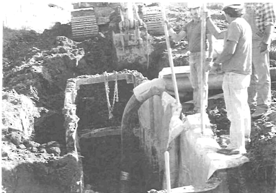
Figure 3 On the north side of this project it was necessary to use a trench box to keep the moisture saturated walls of the trench from collapsing. In this photo, the installation operation is progressing away from the camera. The perforated pipe is being fed through the bottom of the next drain section. When the leading backhoe pulls the trenchbox forward, the men on the right side of the photo will use the sticks with hooks to lower the drain sections under the brace and pull them back into place.
