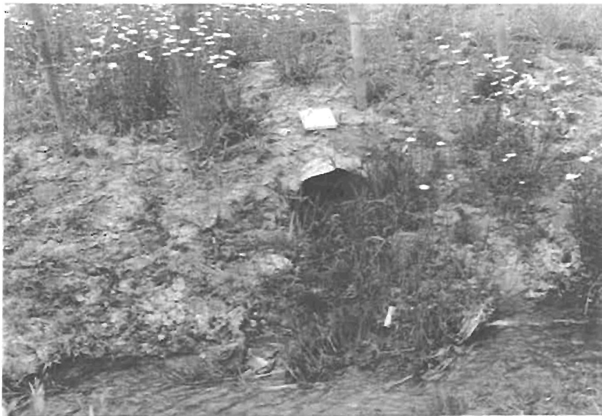
Figure 20 A relatively small amount of water, as seen coming from this pipe on the east side of the roadway, was collected by the system. The most observed was about 20 liters (5.3 gallons) per minute. The water in the foreground is from the roadside ditches and the channel above the curtain drain.
