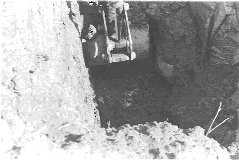
Figure 22 In September of 1990, a section of the drain was excavated with a backhoe and examined. The top of the curtain drain was found at a depth of almost two meters (six feet). The water in this photo at the bottom of the trench is due to the accidental cutting into the perforated pipe.
