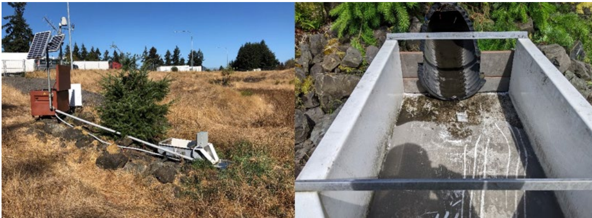
Figure 6 - (Left) Scatter Cr Monitoring Station; (Right) Pipe Outfall to Flume
