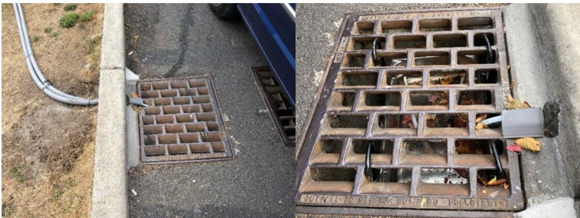
Figure 4 - Sampled Catchbasin with Tubing Connecting to Autosampler (Cleaned Prior to Storm Events)
