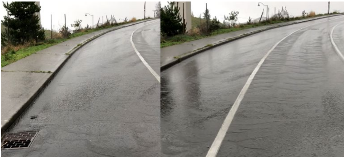
Figure 2 - Eastward Lanes Stormwater Runoff and Receiving Catchbasin
