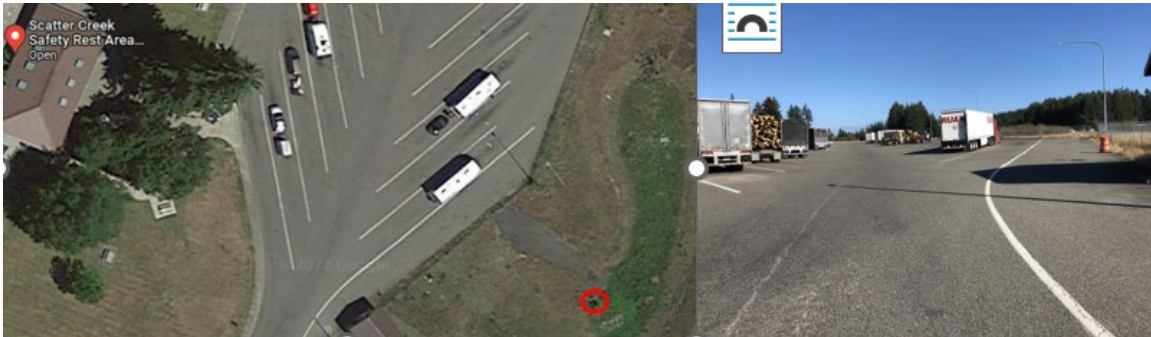
Figure 5 - Scatter Cr Rest Area Northbound Truck Parking/Stormwater Drainage Area
