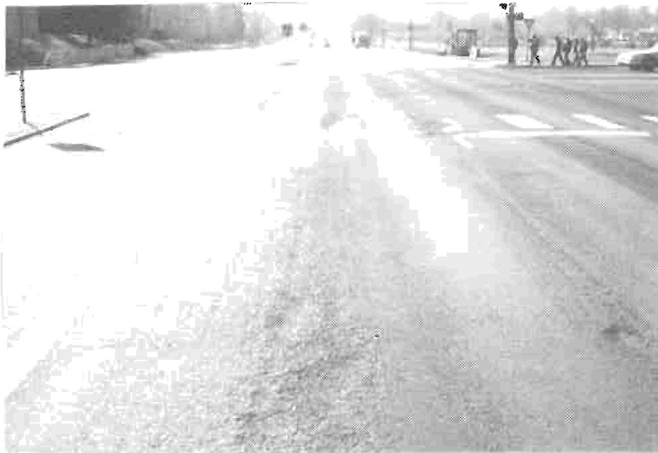
Fig. 1. A "High Maintenance" Mix Experiencing Ravelling After 15 Months.
