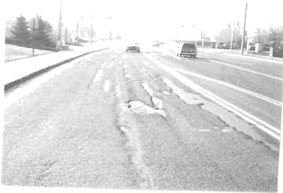
Fig. 5. A Disintegrator After 6 Months.
