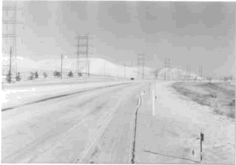
Photograph 3. Test Section 3. 50% Salt + 50% Sand 125 lbs. on Test Section Sunday, January 20, 1991 9:30 A.M.
