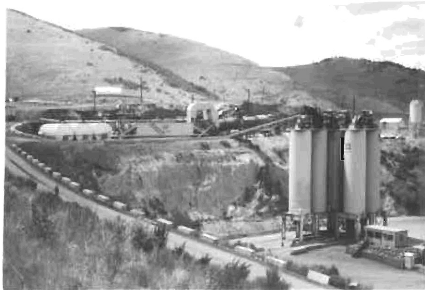
Figure 5. Six, 300-Ton Storage Silos at a Typical Commercial Plant
