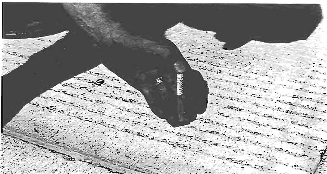
Photo 22: Texture depth measurement using a tire gauge.
