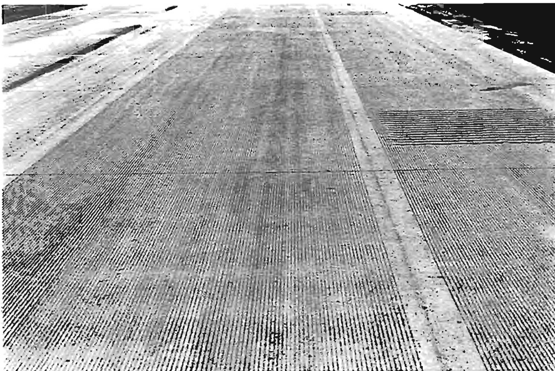
Photo 15: Grooved rumble strip in the right shoulder
