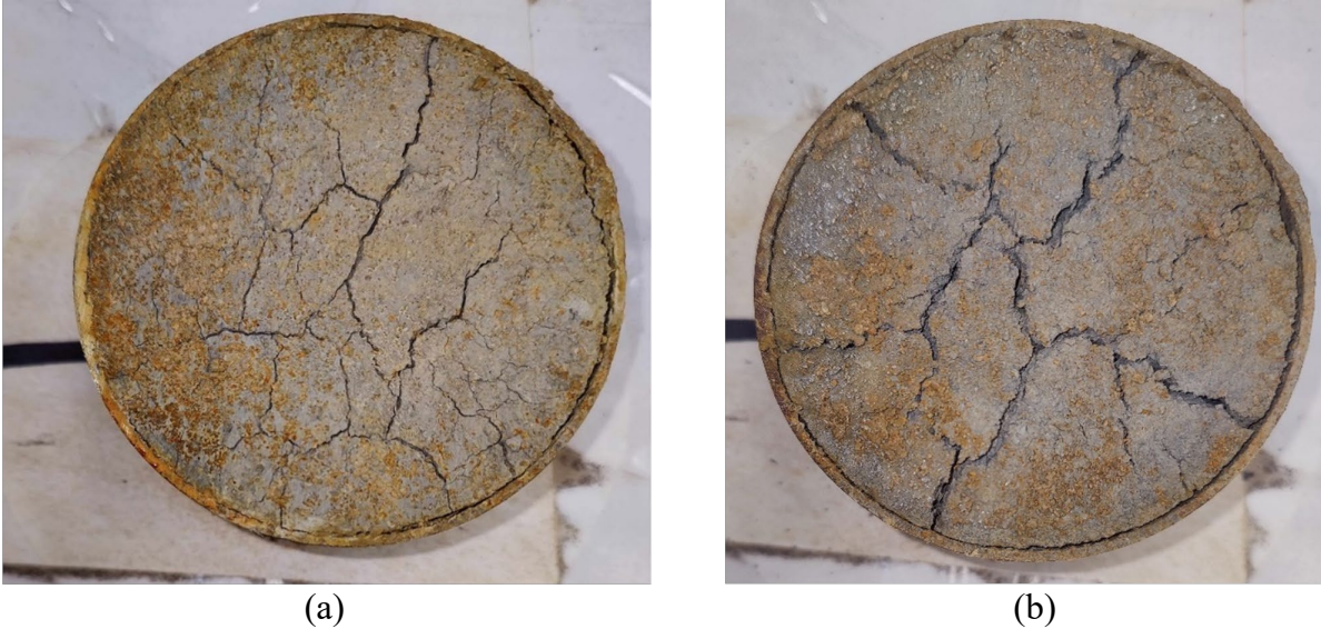
Figure 5.1: Crack Development on Toronto Shale Surface: (a) Surface Crack After 8 th Freeze-Thaw Cycle; (b) Surface Crack After 18 th Freeze-Thaw Cycle
