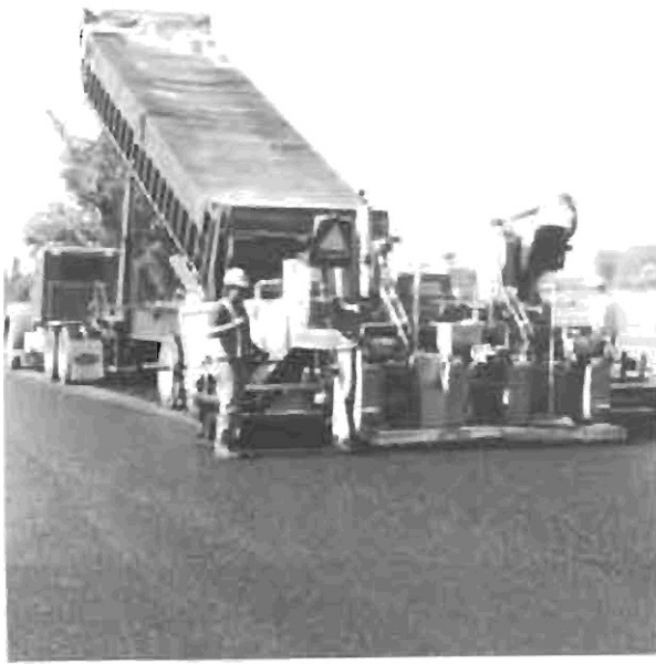
Figure 12. Typical Laydown Operation.
