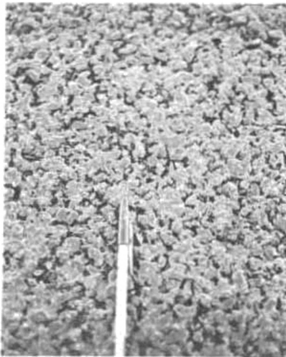
Figure 15. Surface Texture of the Finished Mat.
