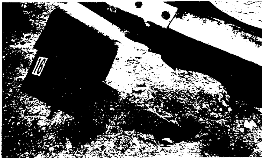
Figure 76. Damage at posts 15 and 16. test 471470-26.
