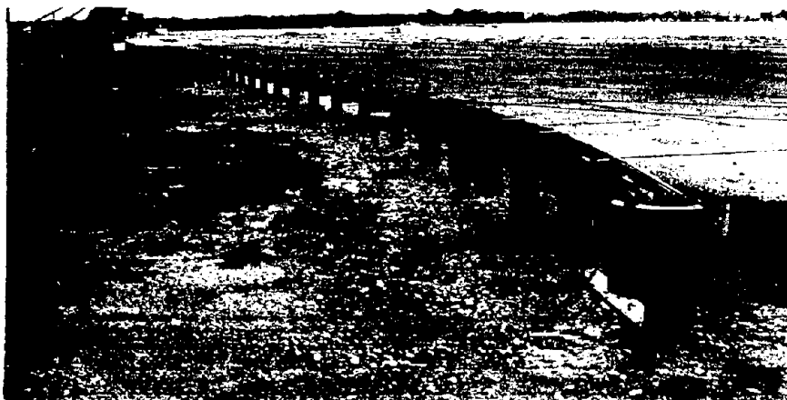
Figure 84. W-beam, steel-post (G4(1S)) guardrail installation before test 471470-27.
