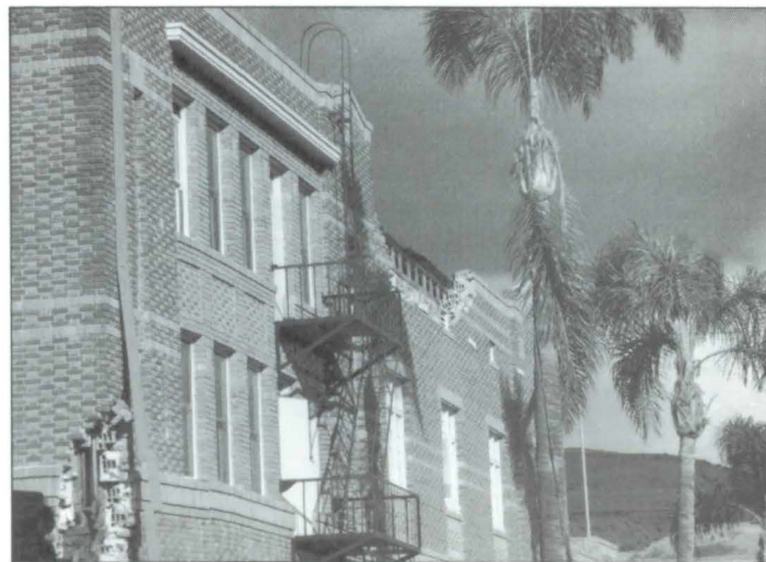
The damaged Masonic Building in Fillmore, California, after the quake.
