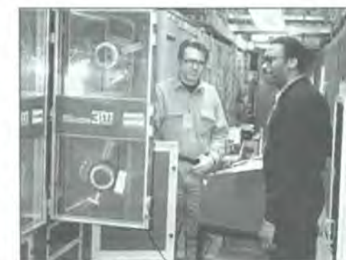
John Szajkowski and Mike Gantt, communications technicians, work on HCVR equipment.
