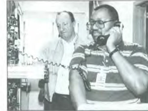
Ralph Humphry and Curtis Alderman make equipment checks at San Jose tower.
