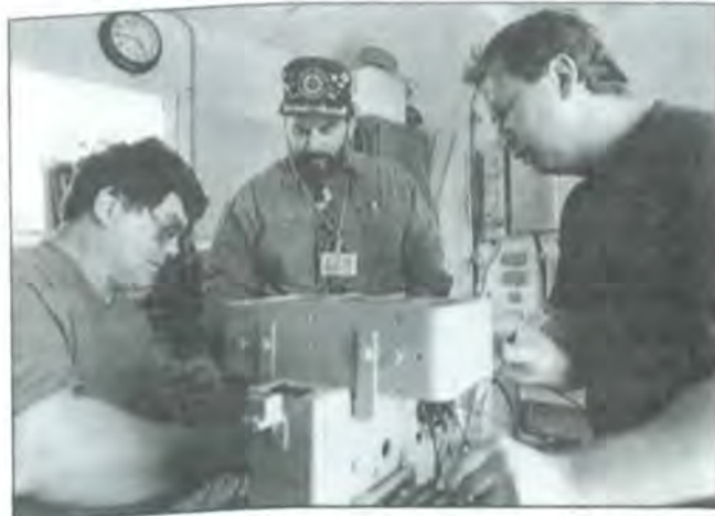
At Atlantic City, environmental unit personnel Wayne King, Ed Irizarry, and Keith Sersen repair approach lights.
