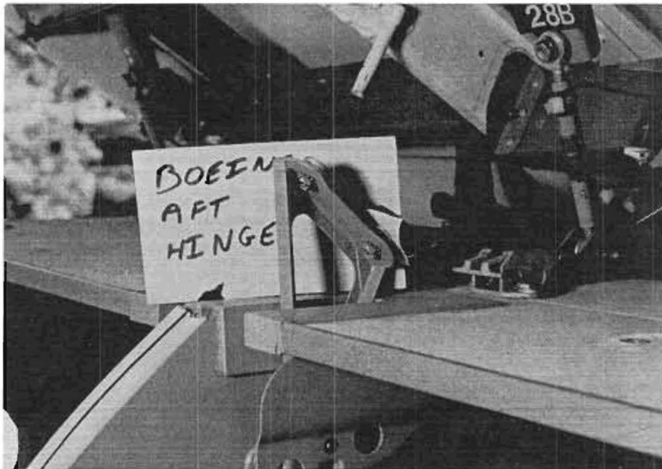
FIGURE 44. BOEING BIN BROKEN AFT HINGE, POSTTEST
